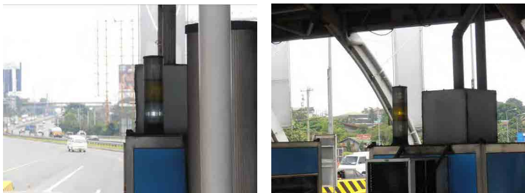
FIGURE 6.2-14 VEHICLE CLASS REPEATER SIGN
