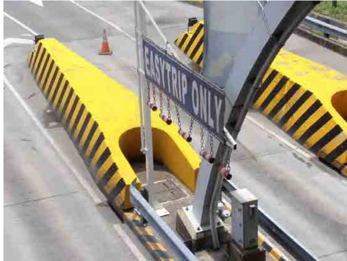
FIGURE 6.2-15 ENTRANCE OF ETC ONLY LANE
