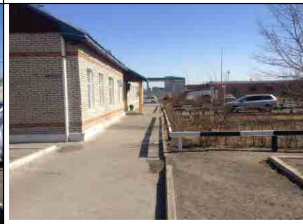
Picture 7: Cement square for pediatric
