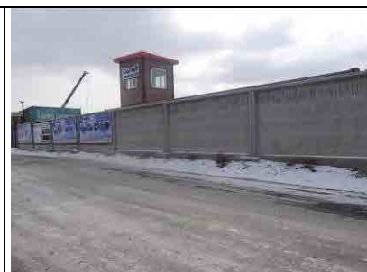
Picture 5: Concrete panels to be relocated
