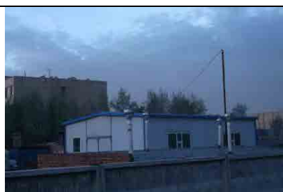
Picture 2: Sandwich warehouse to be relocated
