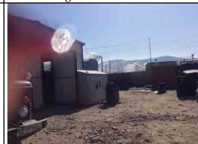
Picture 7: Iron shed to be moved
