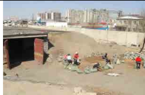
Picture 3: Vegetable storage pit 2 to be relocated
