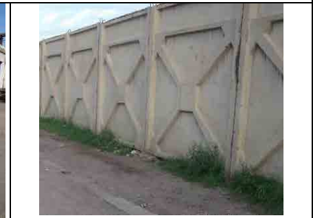
Picture 5: Concrete panels to be moved
