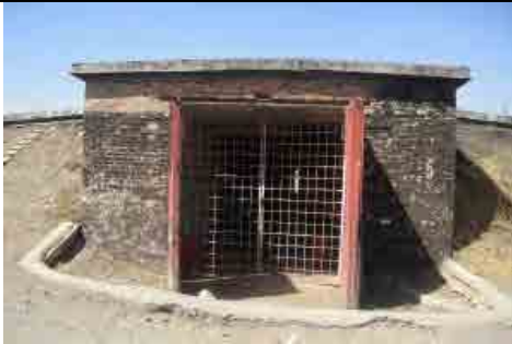
Picture 2: Vegetable storage pit 1 to be relocated
