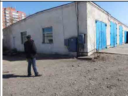
Picture 3: Garage or warehouse to be relocated
