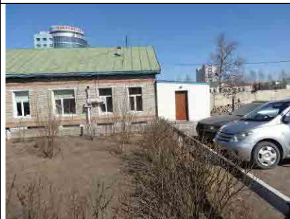
Picture 6: House for toilet and storage with sewerage tank
