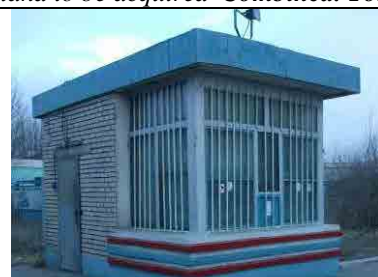
Picture 3: Brick house for guard post of petrol station to be moved
