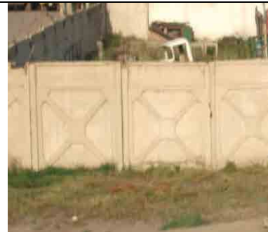
Picture 5: Concrete panels to be moved
