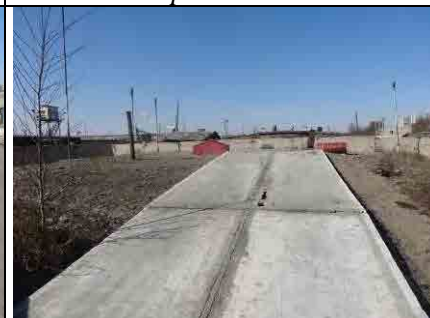
Picture 10: Road to the reservoirs to be moved
