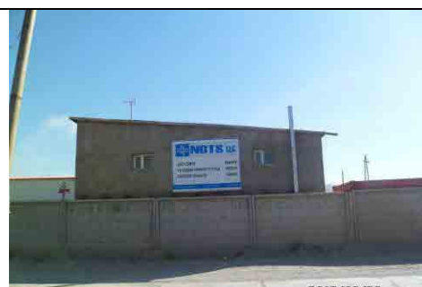
Picture 2: Brick house to be relocated
