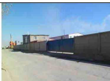
Picture 3: Concrete panels to be relocated
