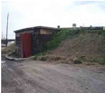
Picture 4: Vegetable storage pit 3 to be relocated
