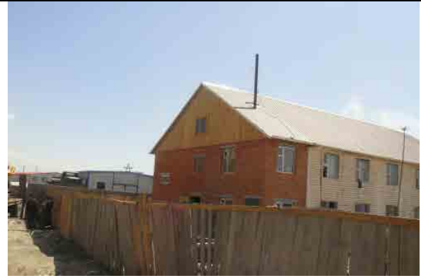
Picture 2: Wooden fence to be relocated
