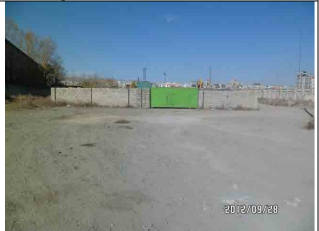
Picture 3: Block wall to be relocated
