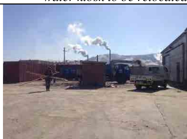
Picture 6: Water kiosk
