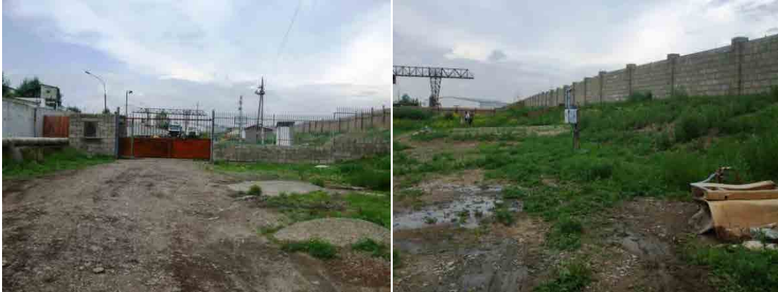
Figure 70. Second location of ground water sampling
