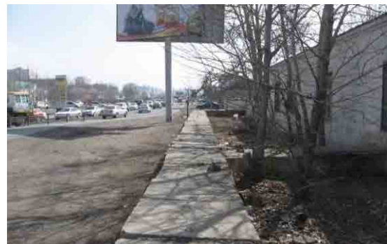
Figure 88. Heat pipeline near STA.1+500
