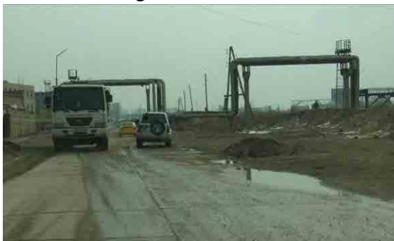
Figure 87. Heat pipeline near STA. 0+440
