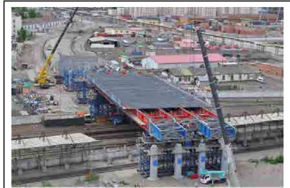
Figure 9.2.4 Launching Erection
