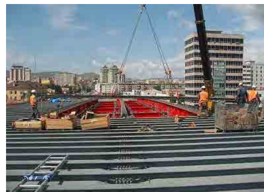
Figure 7.5.5 Construction of Composite Deck Slab
