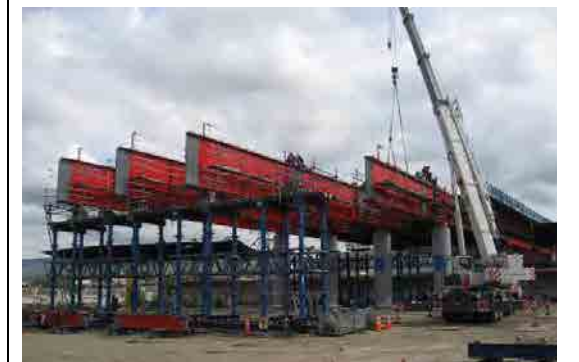
Figure 9.2.5 Crane-Bent Erection
