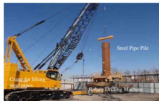
Figure 7.5.1 Construction using Rotary Penetration Steel Pipe Pile
