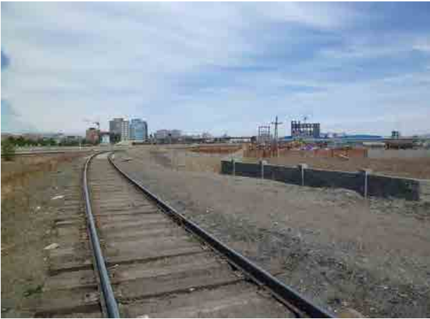
Pic.1 Planned Site of Flyover (1)
