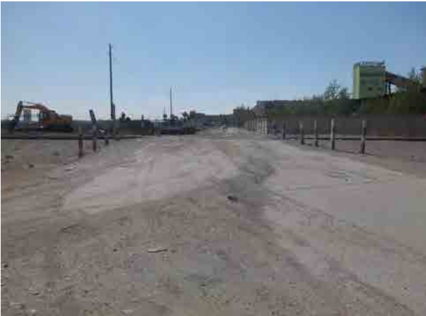
Pic.13 Landing Point near the West Side
