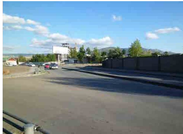
Pic.16 The Place of Grade Separation on Narny Road
