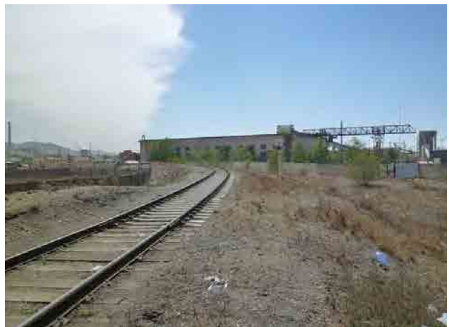
Pic.4 Branch to the Third Thermal Power Plant
