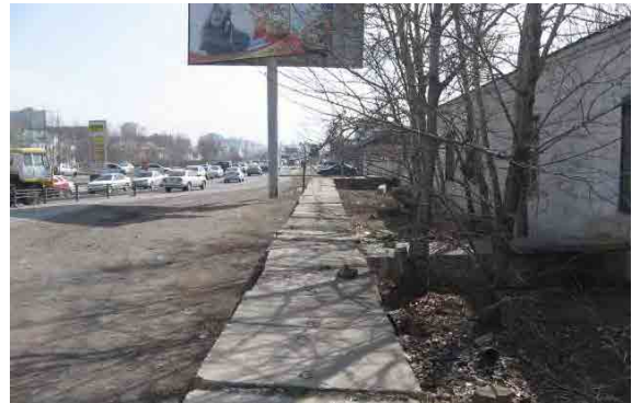
Figure 6.4.4 Hot-Water Pipe around STA. 1+500
