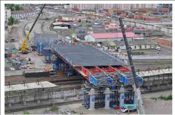
Figure 9.2.4 Launching Erection
