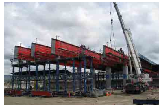
Figure 9.2.5 Crane-Bent Erection
