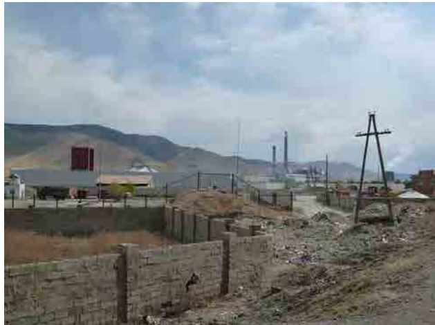
Pic.2 Planned Site of Flyover (2)
