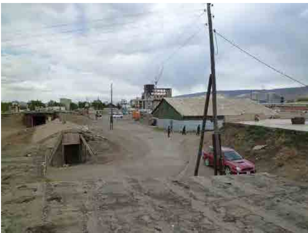
Pic.9 In the Railway facilities (Candidate Site for Material/Equipment Yard)
