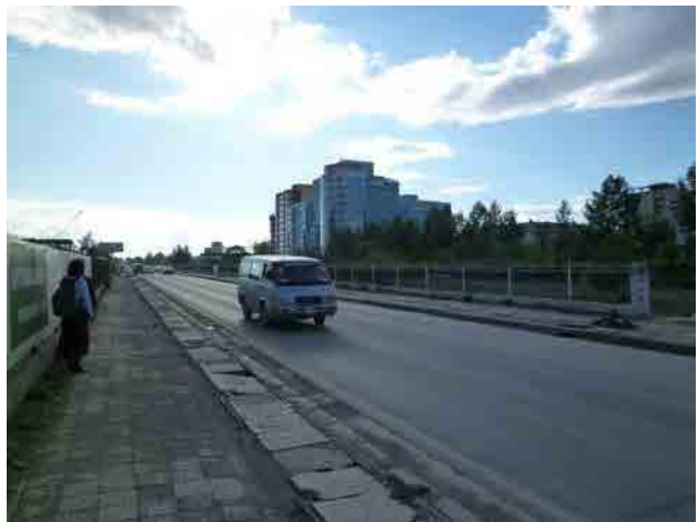
Pic.14 Landing Point near the East Side
