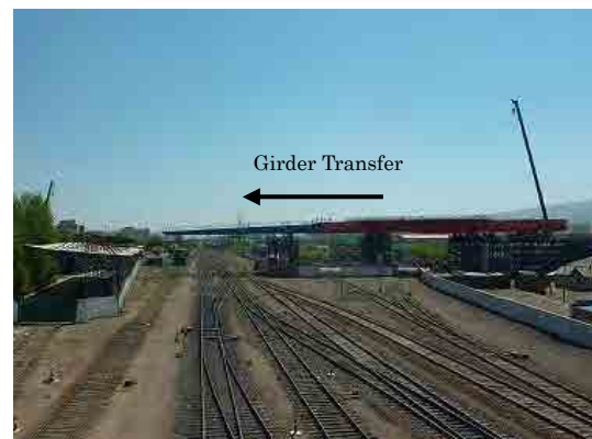
Figure 7.5.8 Erection Method over the Railway Track (Nany Bridge)
