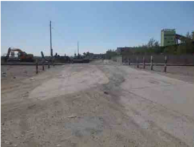
Pic.13 Landing Point near the West Side
