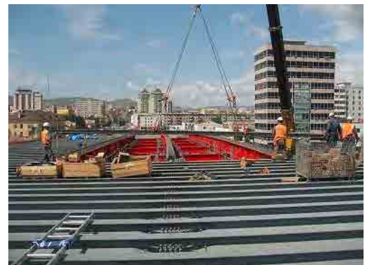
Figure 7.5.5 Construction of Composite Deck Slab
