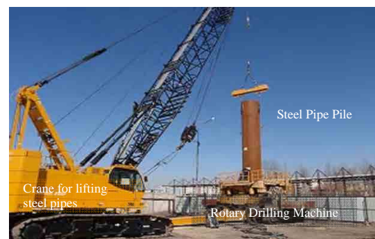
Figure 7.5.1 Construction using Rotary Penetration Steel Pipe Pile
