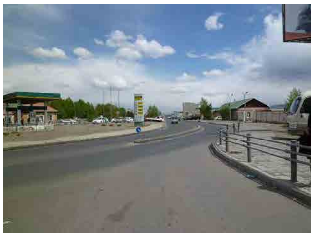
Pic.6 Intersection with Naryn Road (2) (To Ulaanbaatar Station)
