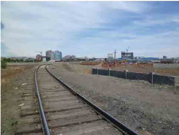
Pic.1 Planned Site of Flyover (1)
