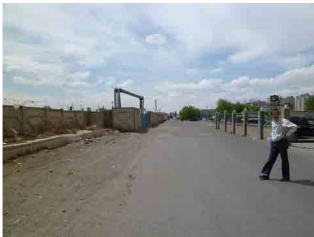
Pic.15 Planned Site of Flyover (Beside of the Railway Facilities)
