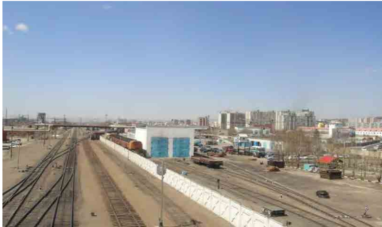
Figure 13. Soil nearby proposed flyover project is naked and compacted
