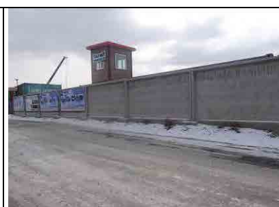
Picture 5: Concrete panels to be relocated
