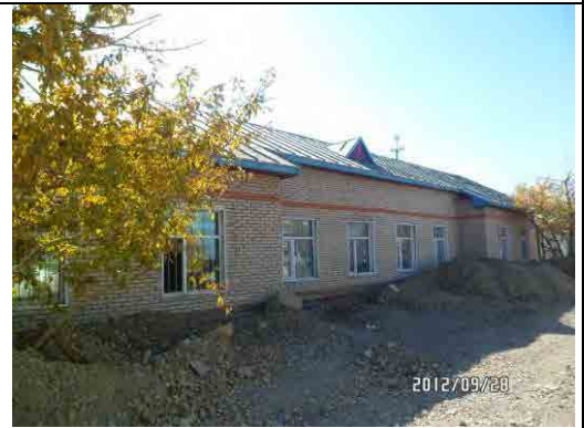
Picture 2: Brick house for staffs` cloak room to be relocated
