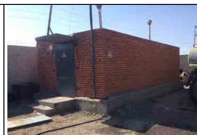
Picture 4: Brick house for generator to be relocated
