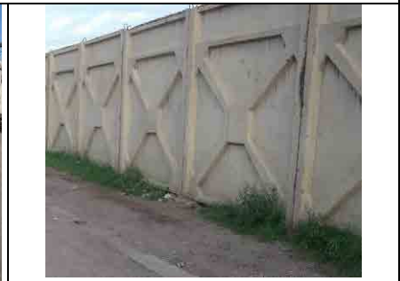
Picture 5: Concrete panels to be moved
