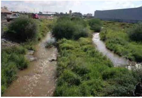
Figure 36. Eastern part of railway of Dund River
