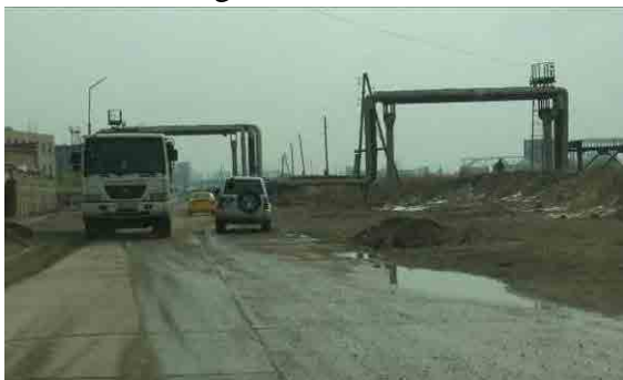
Figure 87. Heat pipeline near STA. 0+440
