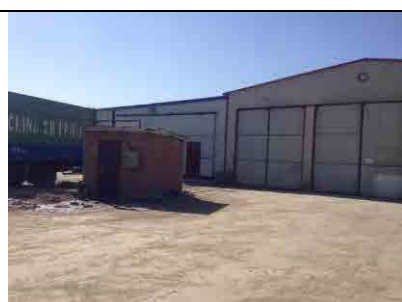
Picture 3: Sandwich structures for office, vacuum window factory and water kiosk to be relocated
