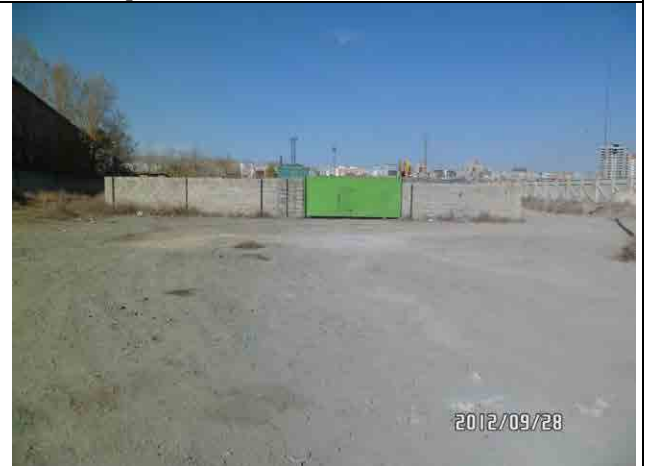
Picture 3: Block wall to be relocated
