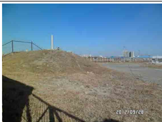
Picture 2: Underground water reserve tank to be relocated
