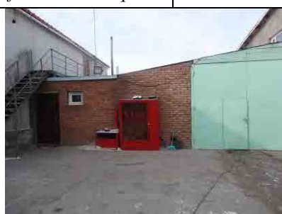
Picture 4: Brick house for toilet and garage to be relocated
