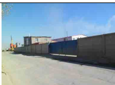
Picture 3: Concrete panels to be relocated
