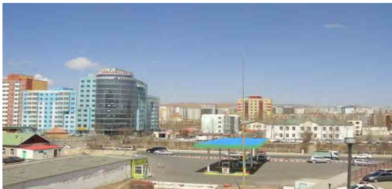
Figure 14. soil nearby proposed flyover project is covered with asphalt road or concrete
