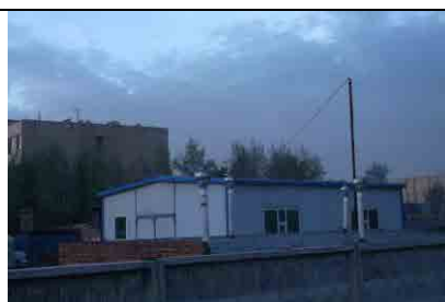
Picture 2: Sandwich warehouse to be relocated
