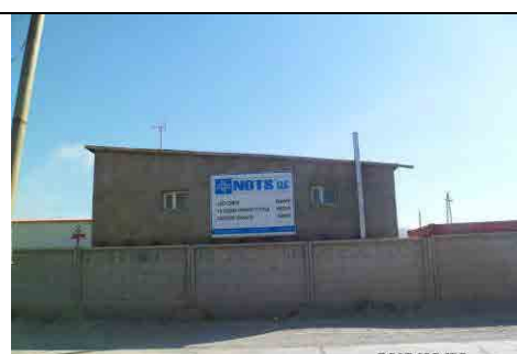
Picture 2: Brick house to be relocated
