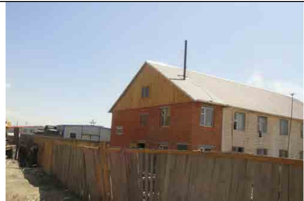
Picture 2: Wooden fence to be relocated
