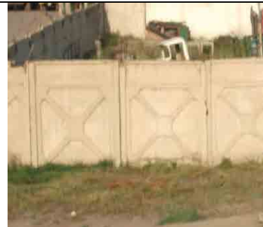
Picture 5: Concrete panels to be moved
