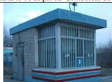
Picture 3: Brick house for guard post of petrol station to be moved
