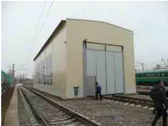
Wheel-tread Grinding Shed
