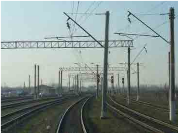
Yard of Marakand Station
