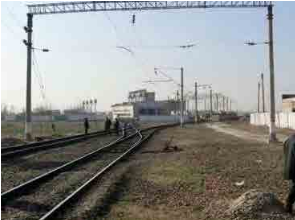
Service Line to Marakand Locomotive Depot
