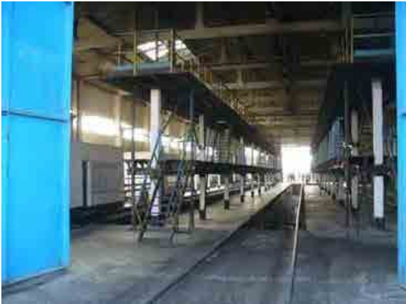
Inside of Inspection and Repair Shed
