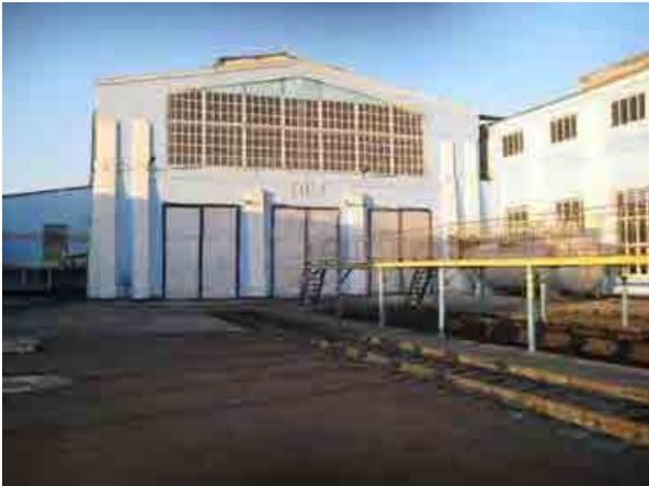
Outside of Inspection and Repair Shed
