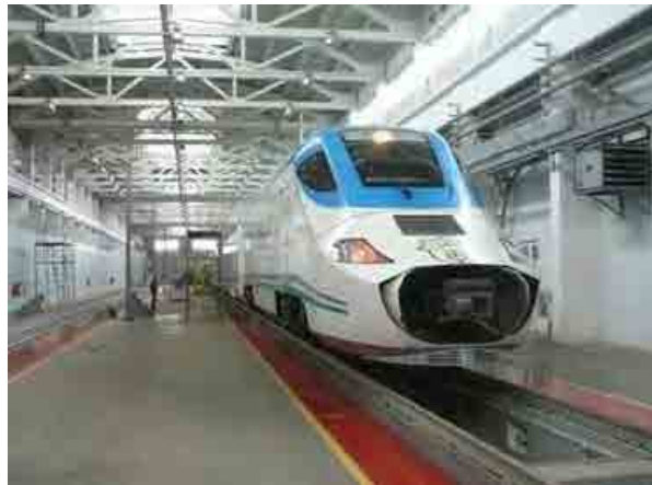
Inside of Inspection and Repair Shed for High-Speed Train "Afrosiyob"
