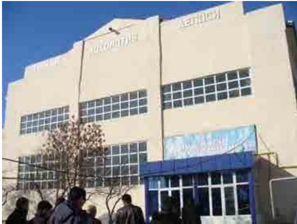
Outside of Existing Inspection and Repair Shed
