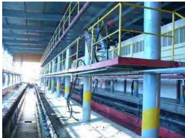
Inside of New Inspection and Repair Shed
