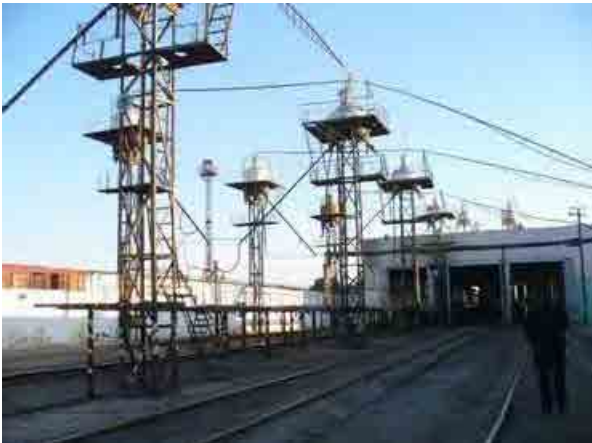
Sand Supply Facility
