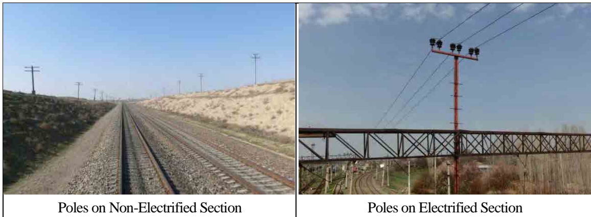
[Pic. 2.4-3] Poles on Non-Electrified and Electrified Sections
