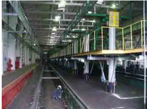
Inside of Inspection and Repair Shed for Electric Locomotive
