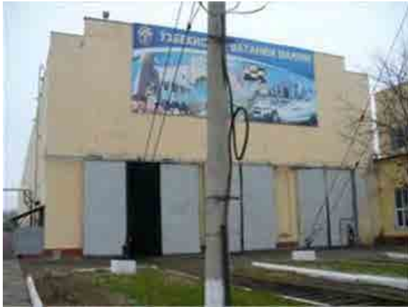
Outside of Inspection and Repair Shed for Electric Locomotive
