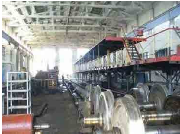
Inside of Existing Inspection and Repair Shed
