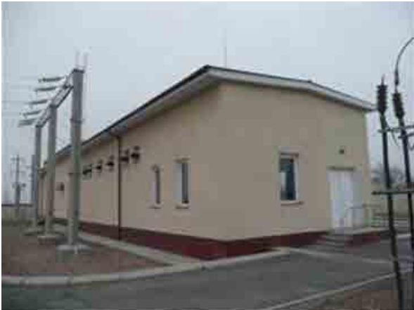
Building of Substation
