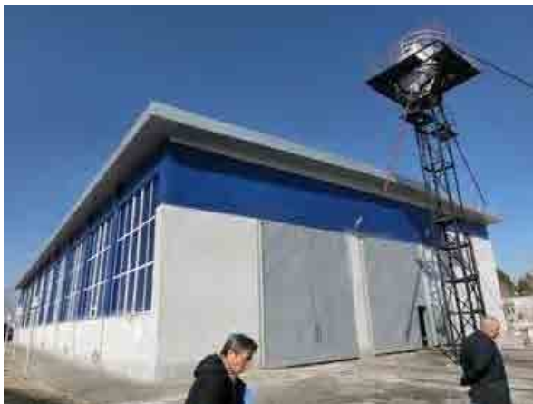
Outside of New Inspection and Repair Shed
