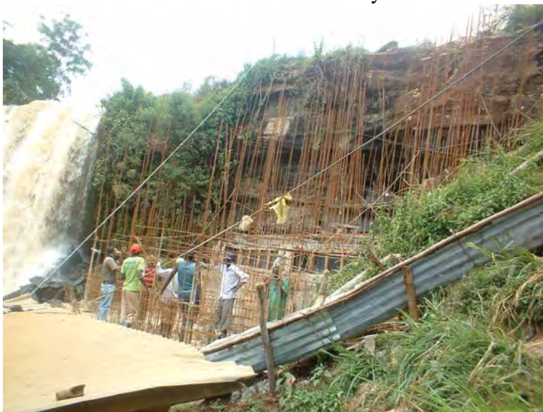
Figure 4.11.4: Site redevelopment Work in progress
