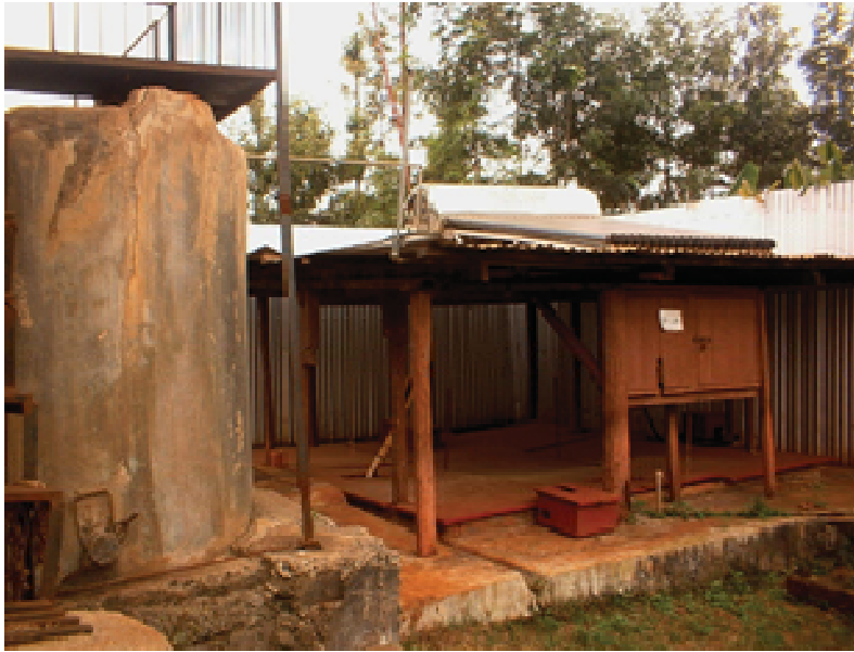
Figure 4.7.2: Kamahuha Biogas Plant
