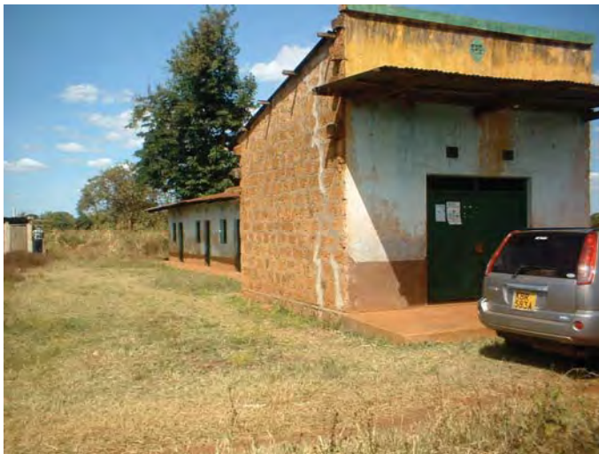
Figure 4.9.1: Makandune CPC Building housing generator and fruits processing machines.
