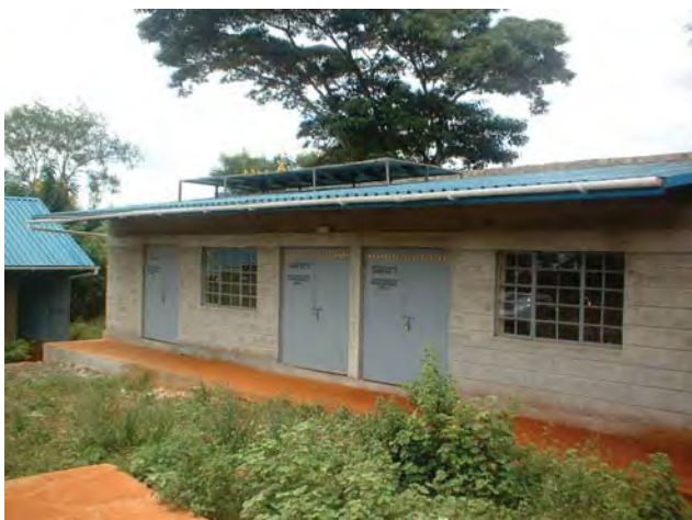
Figure 4.12.2: Kariti Ngando CPC workshop with PV panels on the roof.
