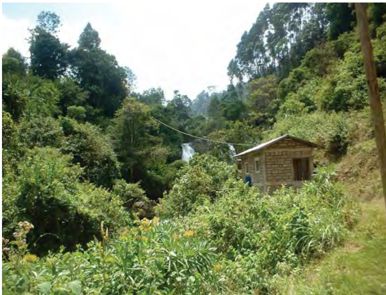
Figure 4.10.1: Mutunguru Microhydro powerhouse
