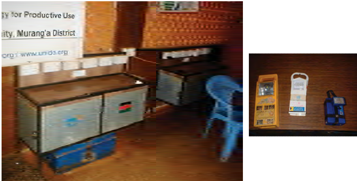
Figure 4.7.7: Charging station. The LED lamps :Accendo, Seco and N-Sunlight make, all from India,
