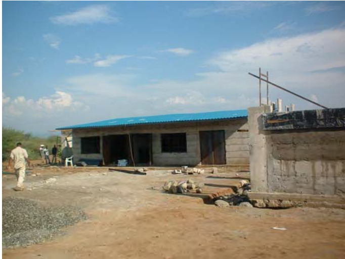
Figure 4.12.5: Civil works in progress at Salaban CPC
