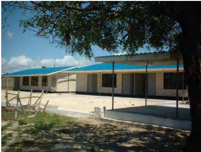
Figure 4.12.3: Rembo Centre CPC Buildings
