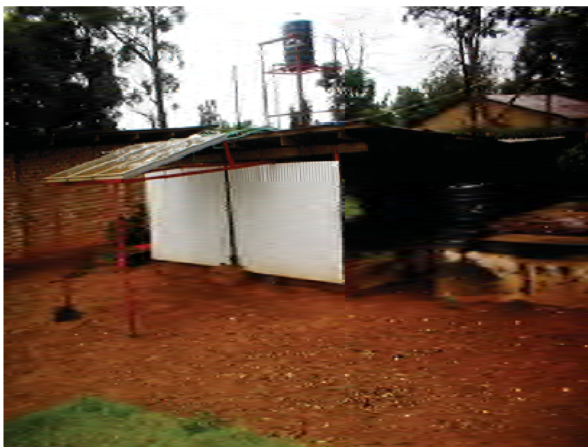
Figure 4.6.1: BMC Biogas Plant
