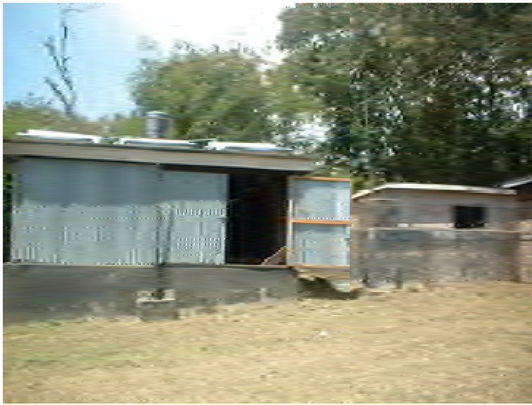
Figure 4.5.5: Biogas Digester – digester tank underground
