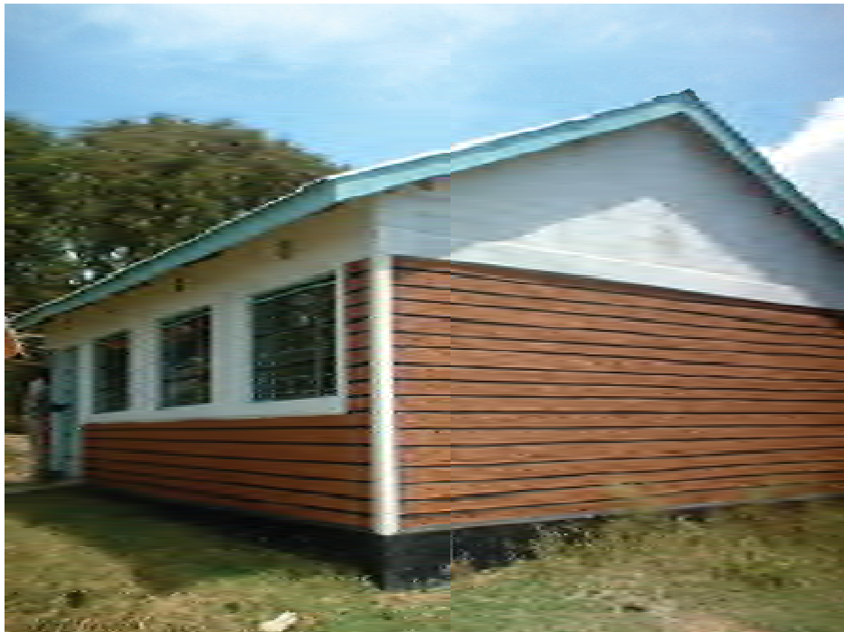
Figure 4.5.8: The Kitchen that has been constructed but not yet equipped
