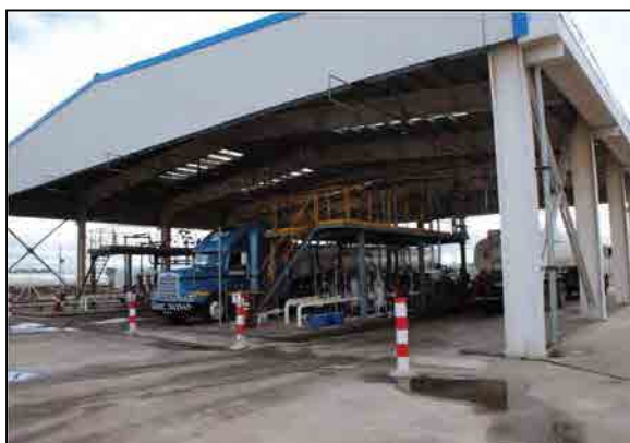
Lorry Unloading Arm
