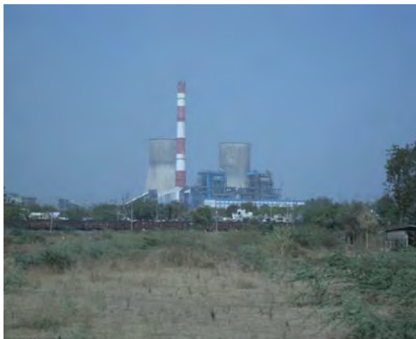
Power Station Overview
