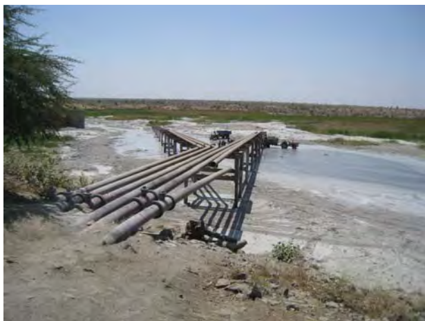
Existing Ash Pond
