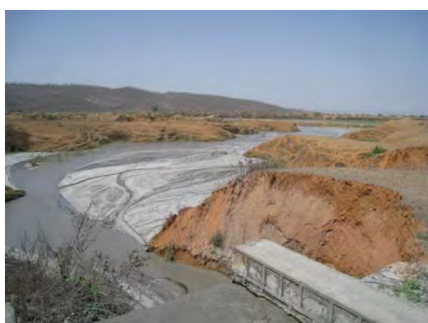
Existing Ash Pond
