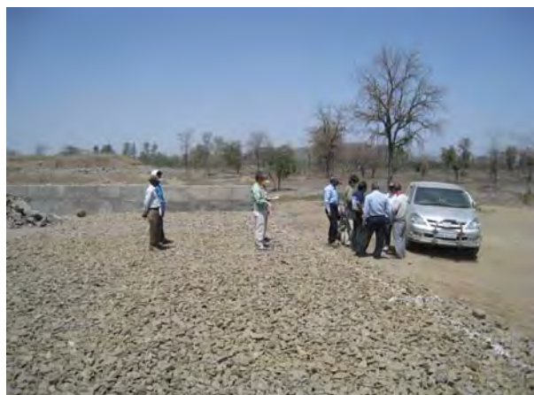
New Ash Pond (under construction)
