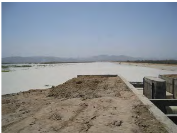
Existing Ash Pond
