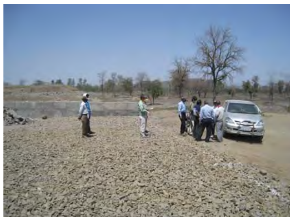
New Ash Pond (under construction)
