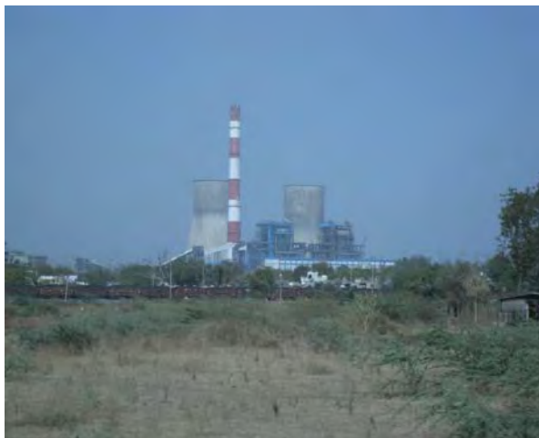
Power Station Overview
