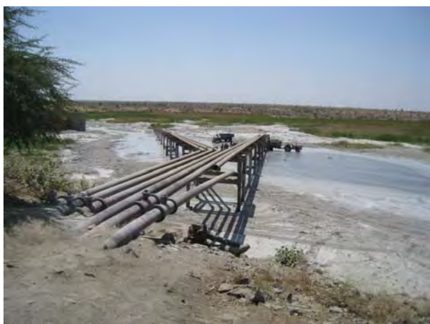
Existing Ash Pond
