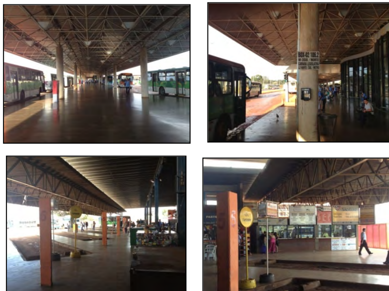
Figure 10-60 Infrastructure of Other Bus Terminals
