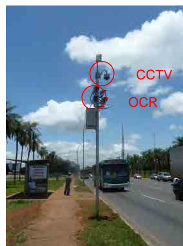
Photo: OCR and CCTV Source: JICA Study Team
