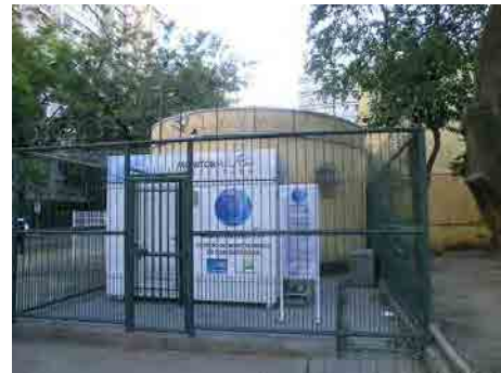
Photo: Monitoring Station (Monitora Rio) Source: JICA Study Team
