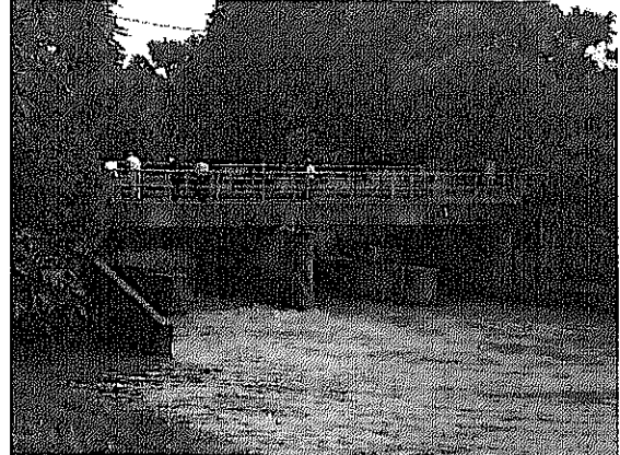
Andong Sla Intake (downstream view)
