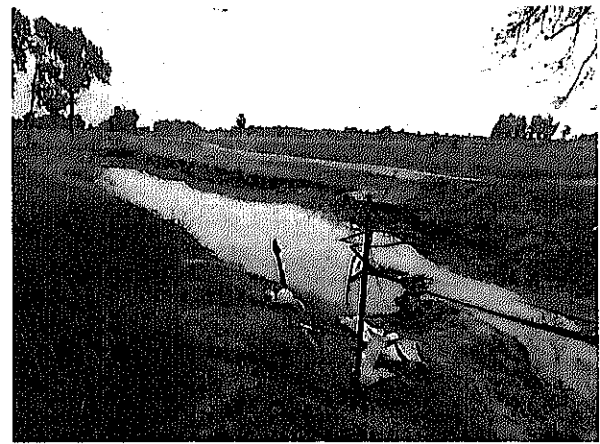
Main canal after recession
