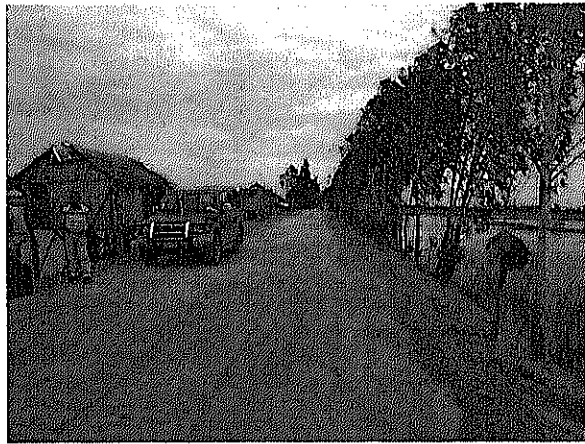
Srass Prambai Reservoir Dike (already rehabilitated)
