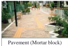
Pavement (Mortar block)
