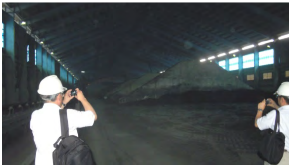
Cement Material Banker (Silica)
