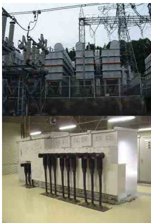
Cubicle for Capacitor Banks (22kV) And Its Cable heads
