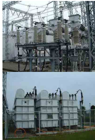
Cable Head For Capacitor Banks (66kV 40MVA)
