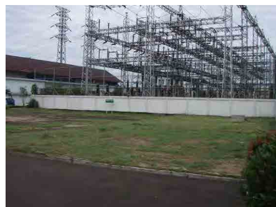
Idle lot of adjacent to Switchyard
