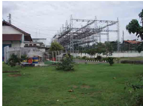
Photo Idle Land of Karet Lama Substation
