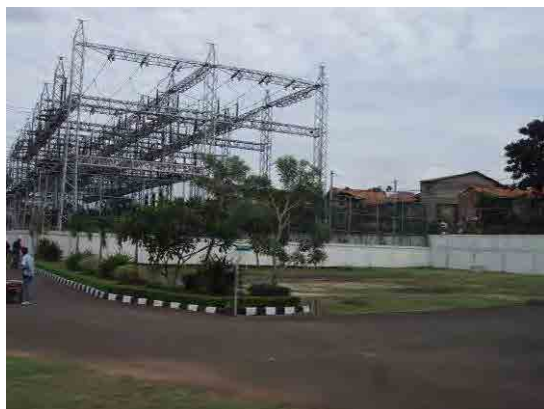
Idle lot of adjacent to Switchyard
