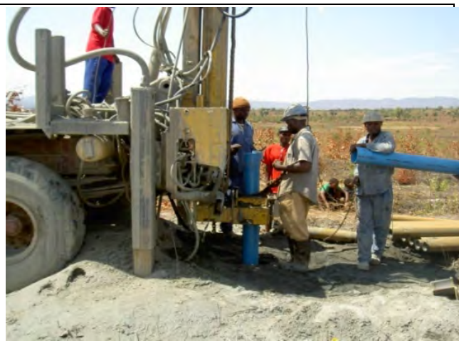
2. Setting of casing (D160mm) at TTC No. 3
