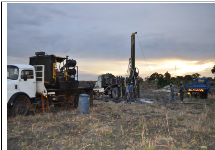
1. Drilling at TTC No. 1
