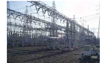
Conventional Air Insulated Substation
