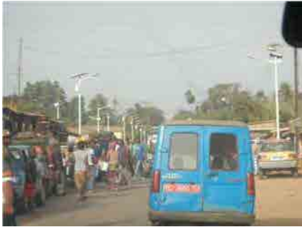
Eclairage routier (Coyah)
