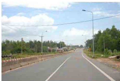
Picture 5.2.16-1 Long Duc Community Road Industrial Zone
