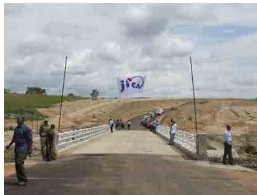
(Completion day: 19th August, 2011)
