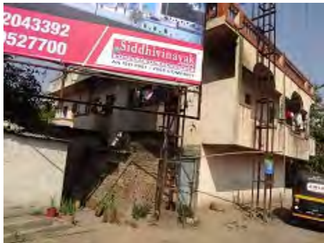
West of NH4 Pic.5: Residence
