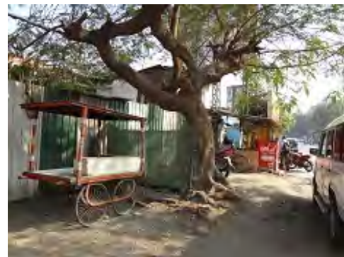
Near Mula river Pic. 4 : Area under construction
