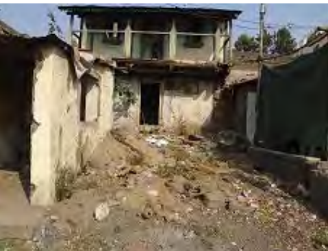
Near Mula river Pic. 15: Residence
