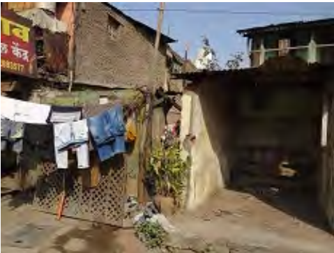
Near Mula river Pic.13: Residence
