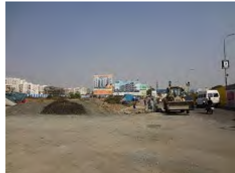
East of NH4 Pic.14: Area under construction
