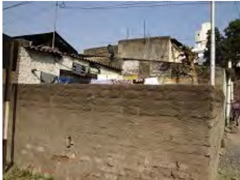
Near Mula river Pic. 20 : Residence
