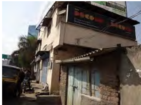
West of NH4 Pic.6: Residence
