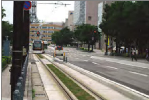
Photo : Toyama Light Rail
