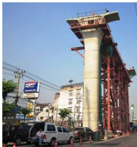
Figure 5.7.1 Image of Construction by Cast-on-stage method
