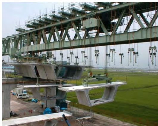
Figure 5.7.3 Image of construction by precast segment method
