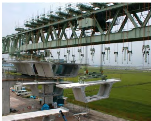
Figure 5.7.3 Image of construction by precast segment method
