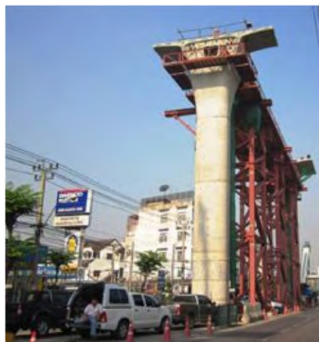
Figure 5.7.1 Image of Construction by Cast-on-stage method
