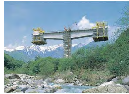
Figure 5.7.5 Image of Cantilever method
