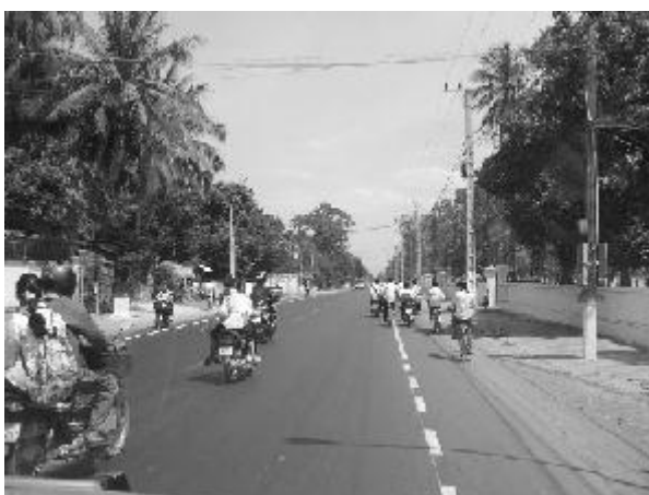
Photo 4.1-1 Edge Line and Paved Shoulder
