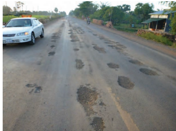
Figure 6 Damaged Pavement
