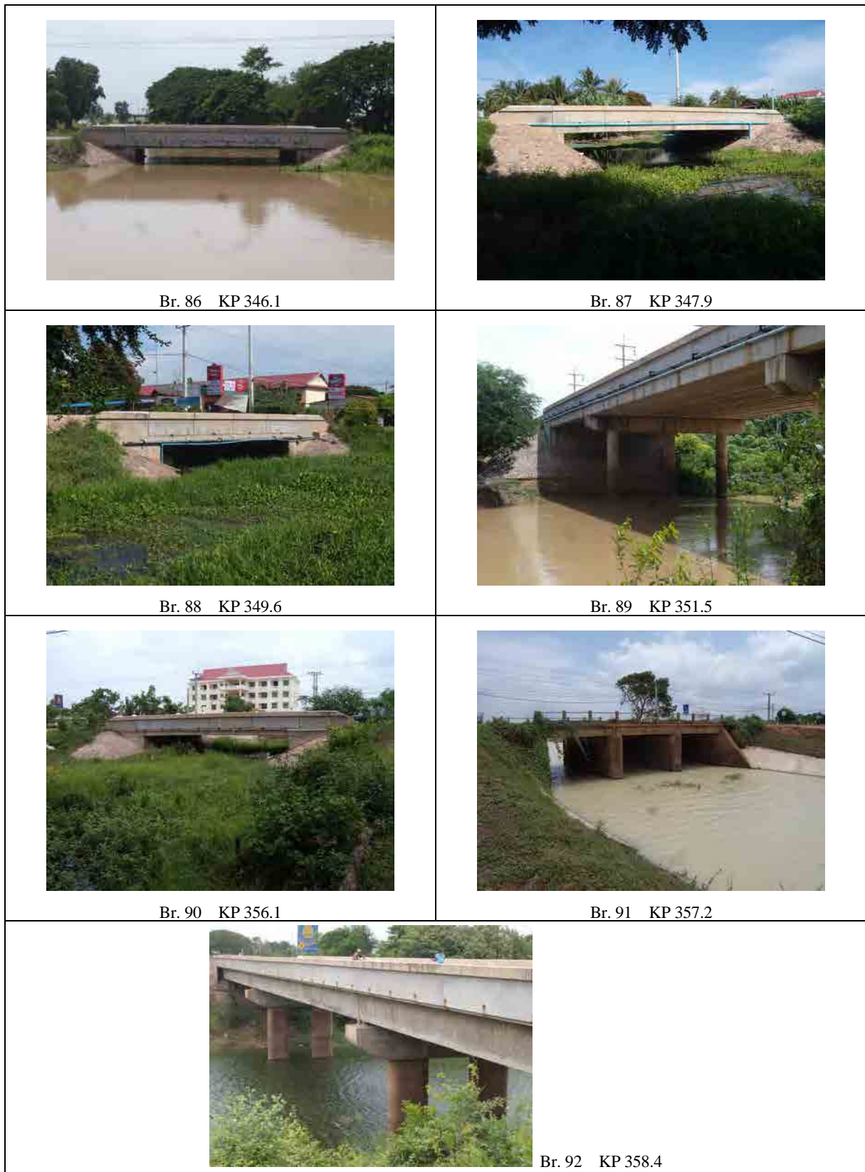
Photo 11.4-2 Existing Bridges on North Section (2/2)
