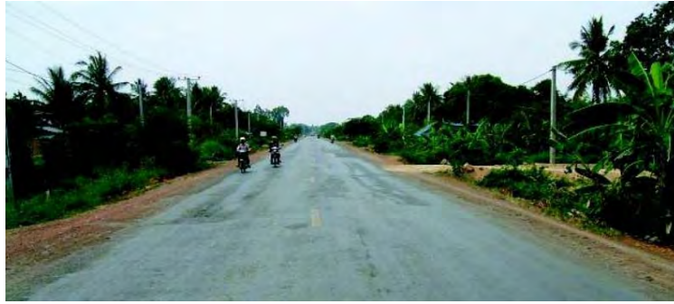
Photo 17.3-1 Sample of Roadside Vegetation along North Section of NR 5
