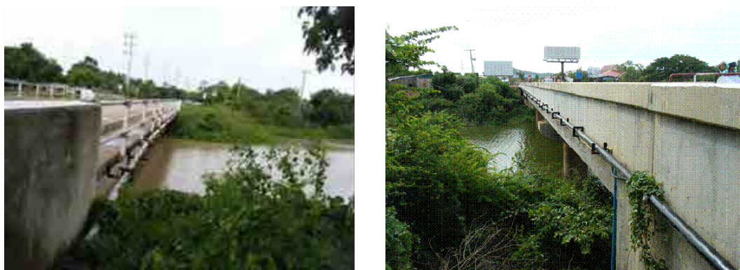
Photo 12.3-1 Utilities at Bridges
