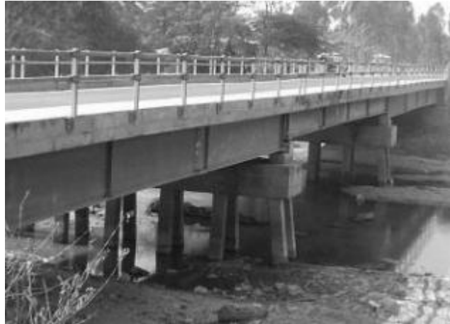
Photo 4.1-4 Battered Piles of Br 26
