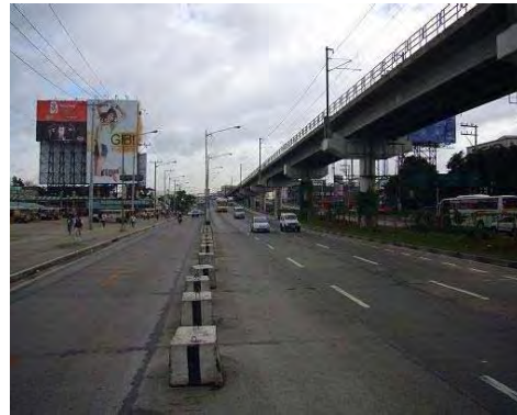
EDSA/Quezon Interchange Flyover along EDSA
