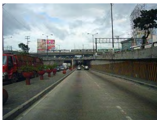
EDS/Quezon Interchange Underpass along Quezon Avenue
