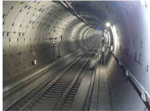
After Excavation Tunnel
