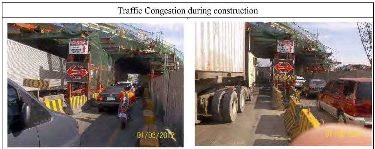
Above picture is shown for shoring/scaffolding of voided slab during construction for similar project. Traffic lane become 2 lanes from existing 3 lanes and cause of heavy traffic jam during construction
