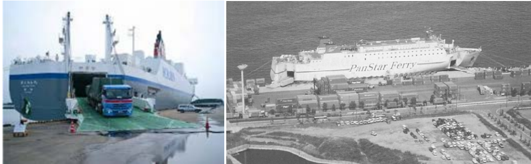
A RO-RO ship with quarter ramps – ships dock alongside quay wall – this type of RO-RO ships is capable of docking at a general berth without a dedicated shore facility for vehicle
