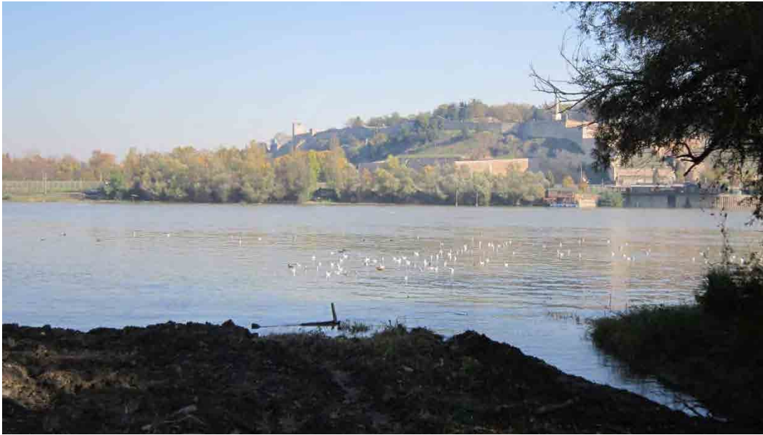
Figure 9. Location of the wastewater outflow via the Usce pumping station and the location of where Interceptor No. 1 will cross the Sava River. The Belgrade Fortress can be seen in the background.
