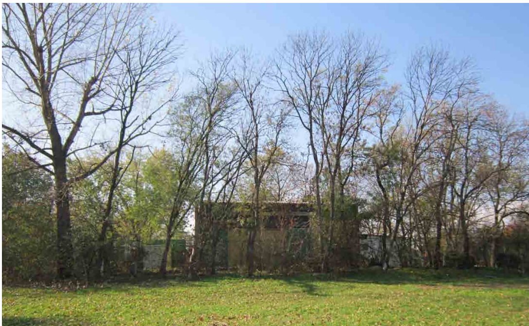
Figure 10. The existing Usce pumping station
