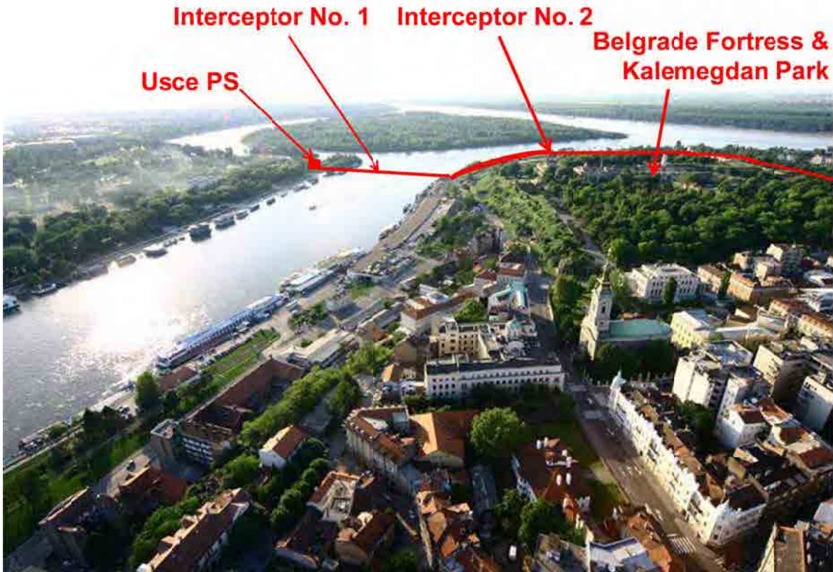
Figure 8. General layout plan showing the location of Usce PS, Interceptors 1 and 2 and the surrounding area – the Usce Park around the Usce PS and the Belgrade.
