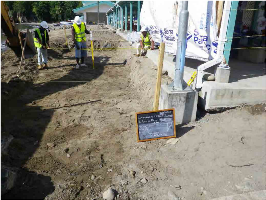
Around No.0 Digging
