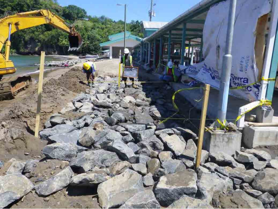
Around No.0 Laying of rubble stones
