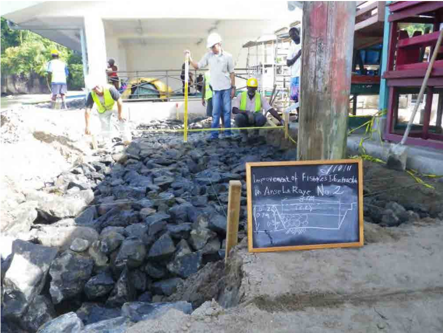
Around No.2 Laying of rubble stones
