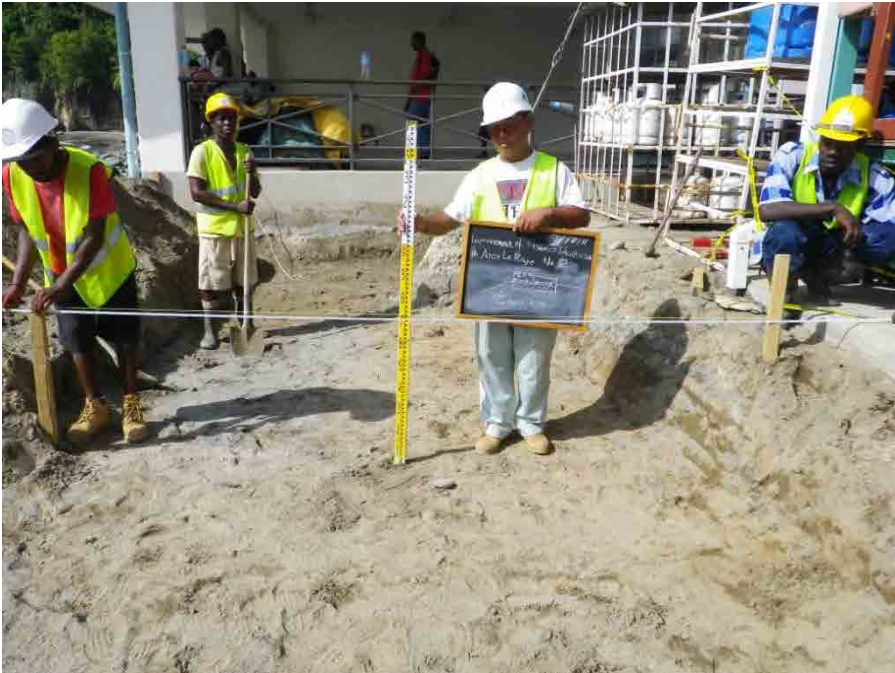
Around No.2 Completion of digging
