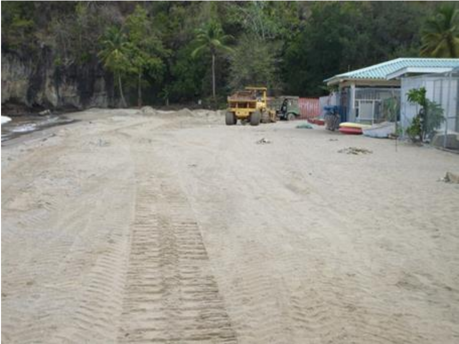
Photo 5-3-2-1 Completion of protection of Fishing Gear Lockers
