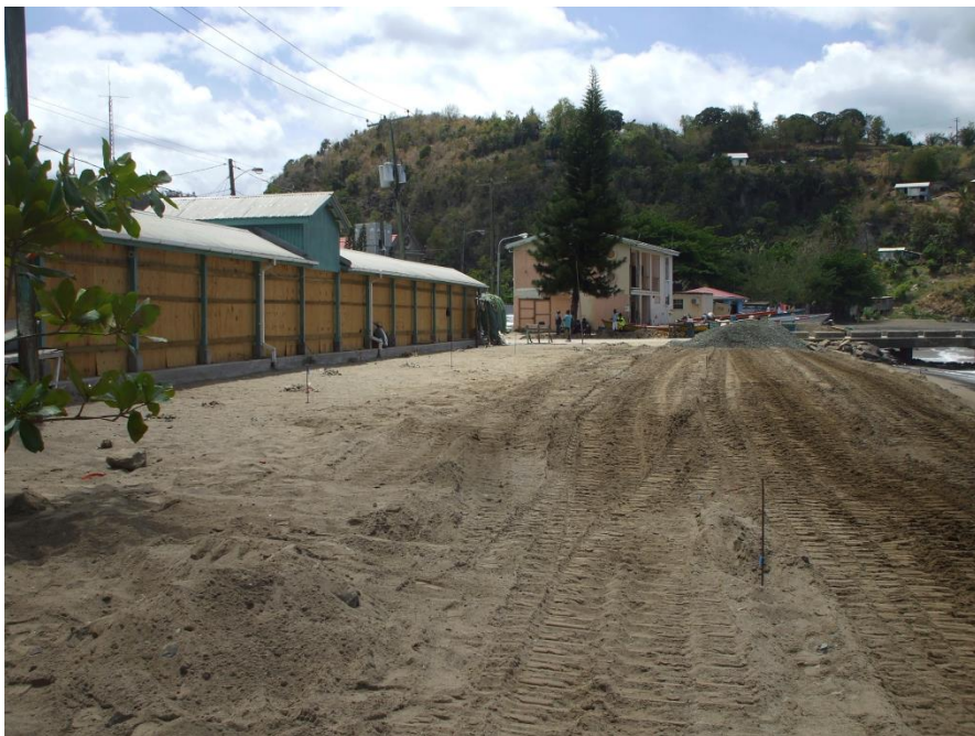
Photo 5-3-2-4 Completion of protection of Vendors Arcade
