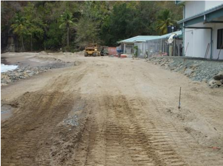
Photo 5-3-2-2 Completion of protection of Fisheries Complex (1)
