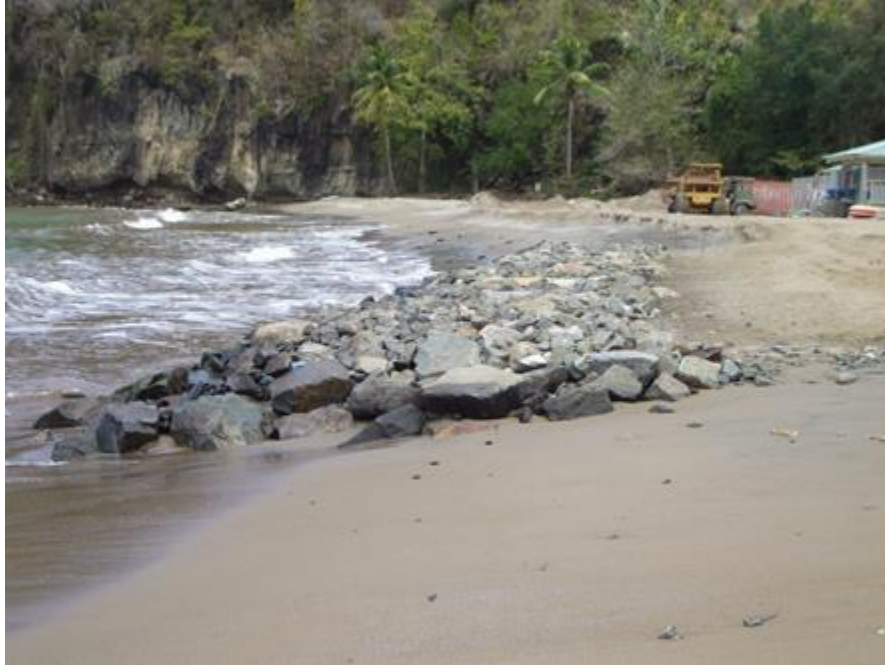
Photo 5-3-2-3 Completion of protection of Fisheries Complex (2)
