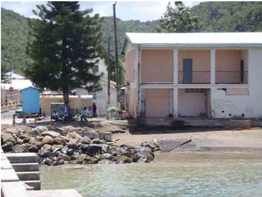
Photo 2-2-3-7 Foreshore status before execution of short-term countermeasure works
