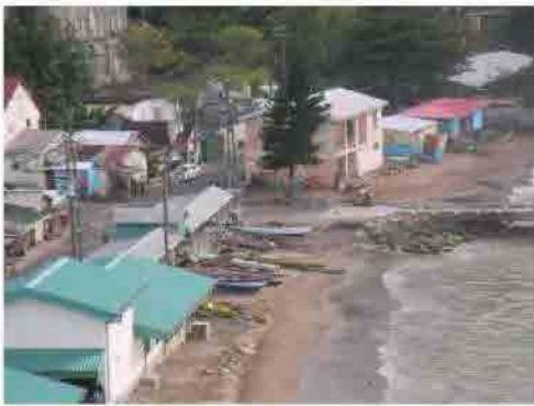
Subsidence and recession of shoreline in front of Vendors Arcade
