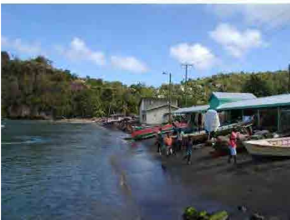
Photo-5 Foreshore condition of Vendors Arcade at Basic Design (2006/10/20)
