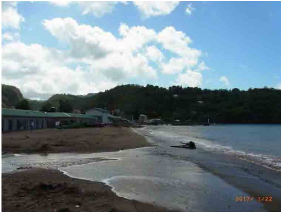
Photo 2-2-3-20 Backshore situation in front of Fishing Gear Lockers to Work Shop
