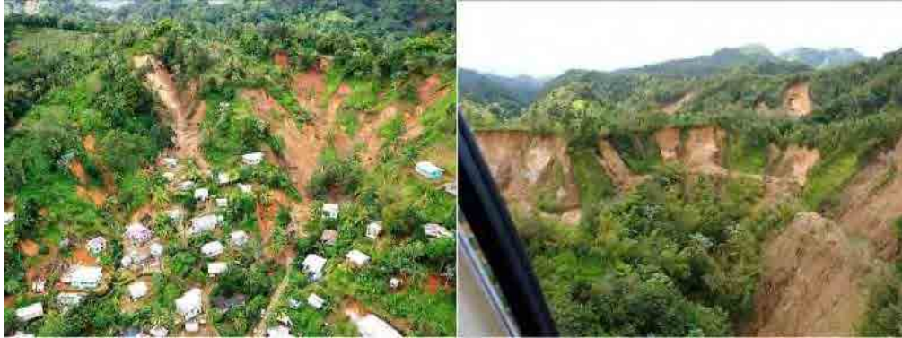
Figure 3-2-3-3 Large scale hillside landslides (Hurricane Tomas)
