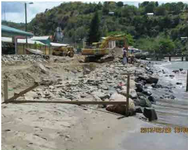
Photo-31 Covering of rubble stones at shoreline in front of Fisheries Complex (2013/2/28)
