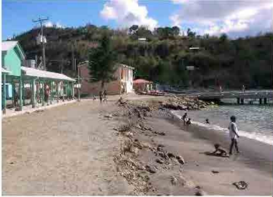
Beach situation in front of Vendors Arcade at completion of construction; Feb. 19, 2010
