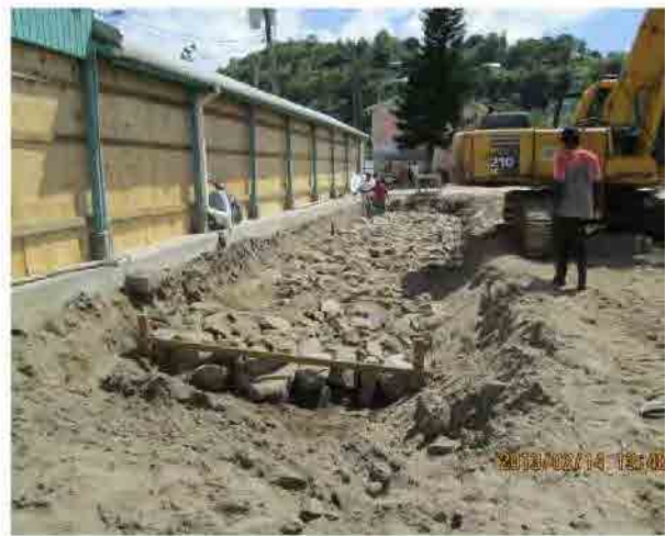
Photo-32 Recovering of rubble stones in front of Vendors Arcade (2013/2/14)
