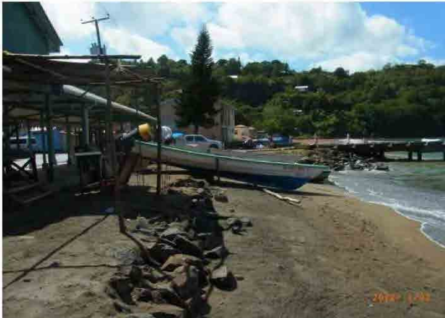
Photo 2-2-3-13 Exposed situation of armor stones
