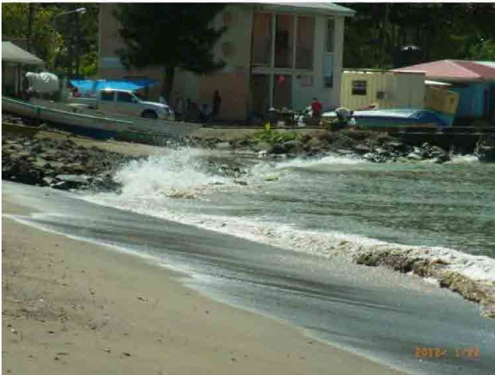
Photo 2-2-3-15 Armor stone part and foreshore slope in front of Fisheries Complex (2)
