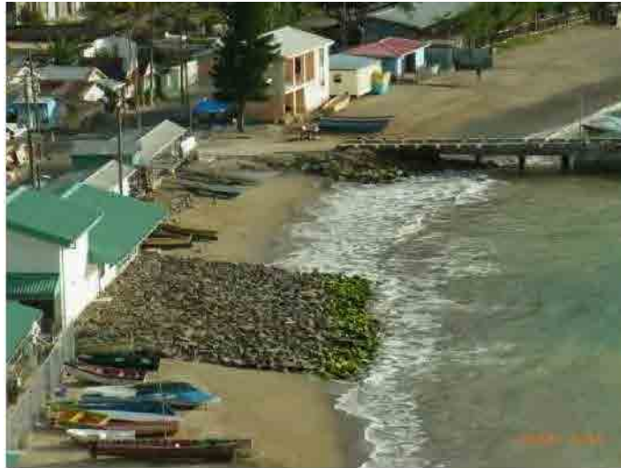
Photo 2-2-3-2 Situation of short-term countermeasure works
