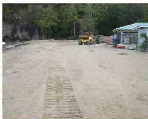
Photo-34 Completion of protection of Fishing Gear Lockers (2013/3/15)
