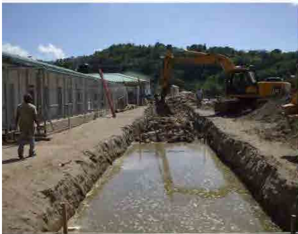
Photo-25 Covering of rubble stones in front of Fishing Gear Lockers (2013/2/1)
