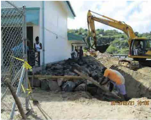
Photo-29 Levering of rubble stones on the foot of Fisheries Complex (2013/2/21)
