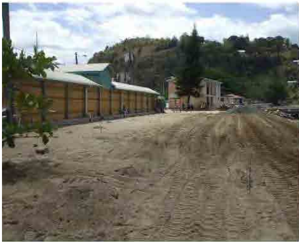
Photo-37 Completion of protection of Vendors Arcade (3015/3/15)
