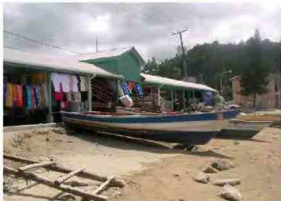
Beach situation in front of Vendors Arcade at one year inspection; Feb. 08, 2011
