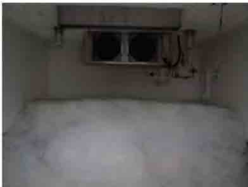
Ice strage room
