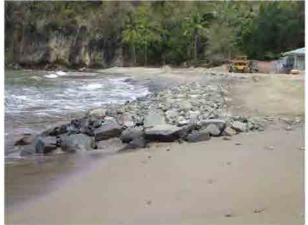
Photo-36 Completion of protection of Fisheries Complex (2) (2013/3/15)
