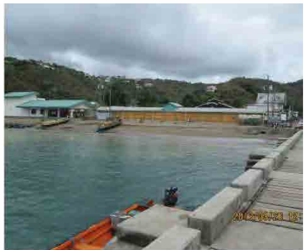
Photo-40 Panoramic view at completion (Foreshore in front of Vendors Arcade) (2013/3/20)
