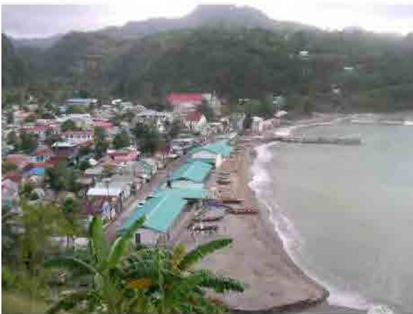
Photo-3 Panoramic view of one year inspection (2011/02/08)
