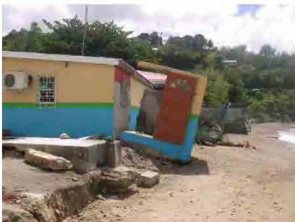
Photo-11 Storehouse of old office of Cooperative (2011/02/28)
