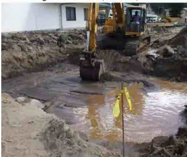
Photo-27 Demolish of rubble stones in front of Fisheries Complex (2013/2/20)
