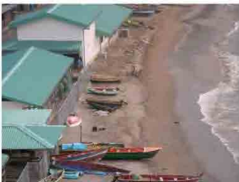
Subsidence and recession of shoreline between Fisheries Complex and the Jetty
