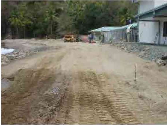
Photo-35 Completion of protection of Fisheries Complex (1) (2013/3/15)
