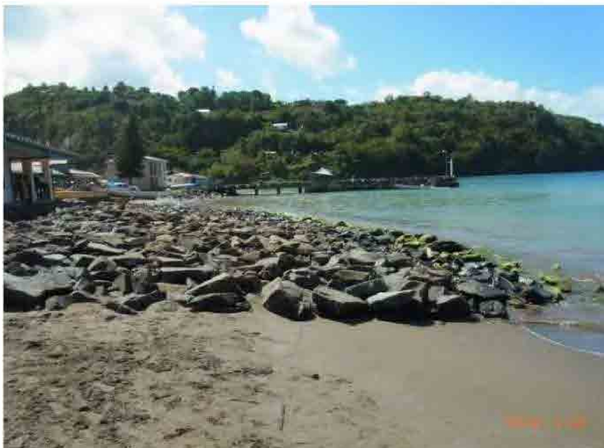
Photo 2-2-3-17 Deposited situation of foreshore at north side of armor stones
