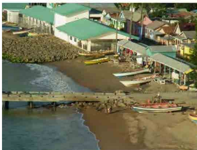
Photo 2-2-3-4 Recovery status at south side of the jetty
