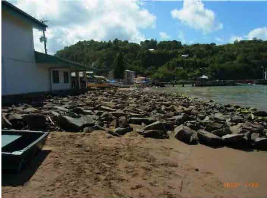
Photo 2-2-3-18 Backshore situation at north side of armor stone part
