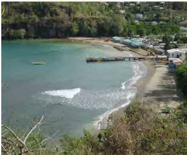
Photo-39 Panoramic view at completion (South side beach) (2013/3/15)
