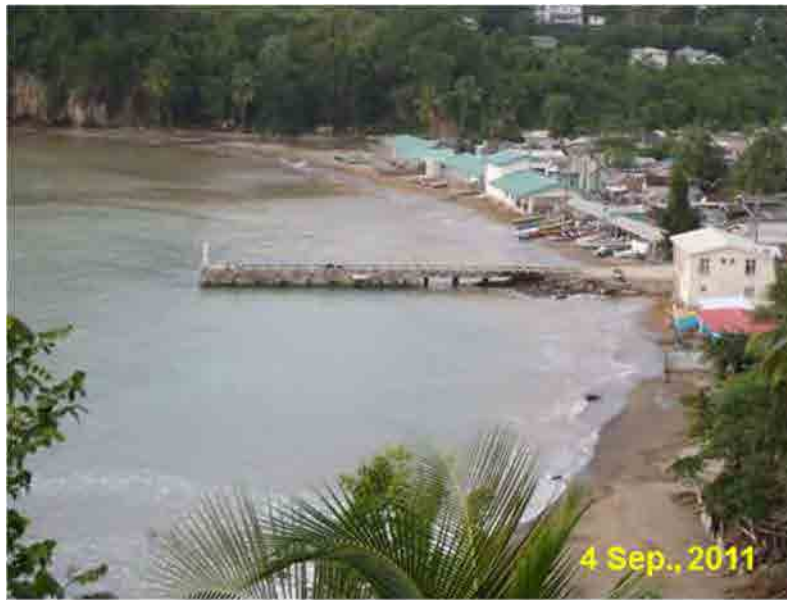
Photo 2-2-3-5 Beach status before short-term countermeasure works
