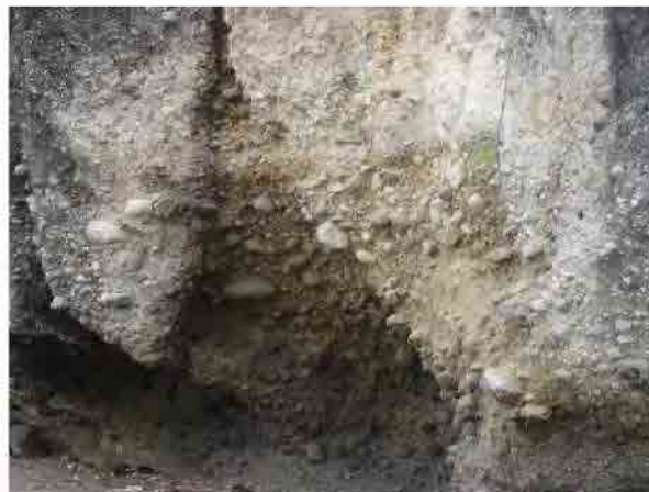
Figure 3-1-2-3 Enlarged photo of coastal cliff
