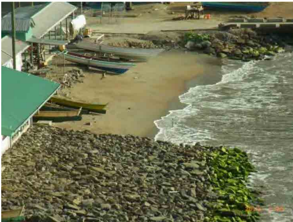
Photo 2-2-3-9 Foreshore situation in front of Vendors Arcade
