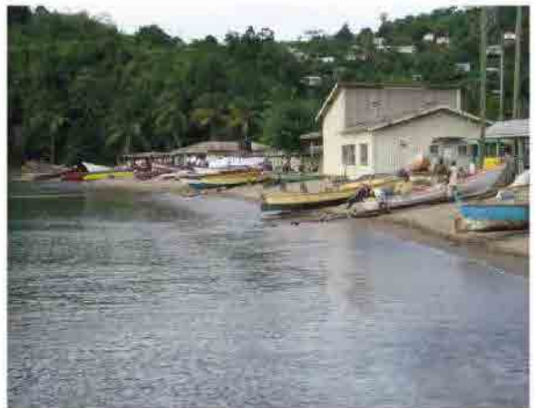
Photo-4 Foreshore condition of Fisheries Complex at Basic Design (2006/10/20)
