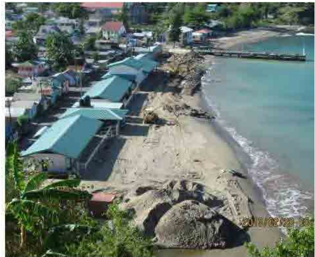
Photo-24 Condition of construction of middle-term countermeasure (2013/2/28)
