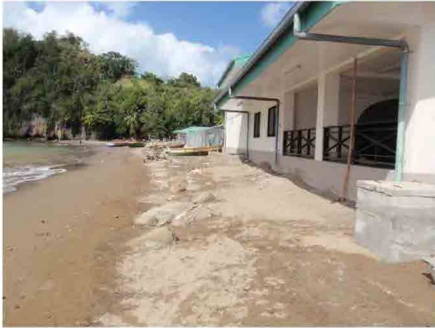
Feb. 08, 2011 at One year inspection
