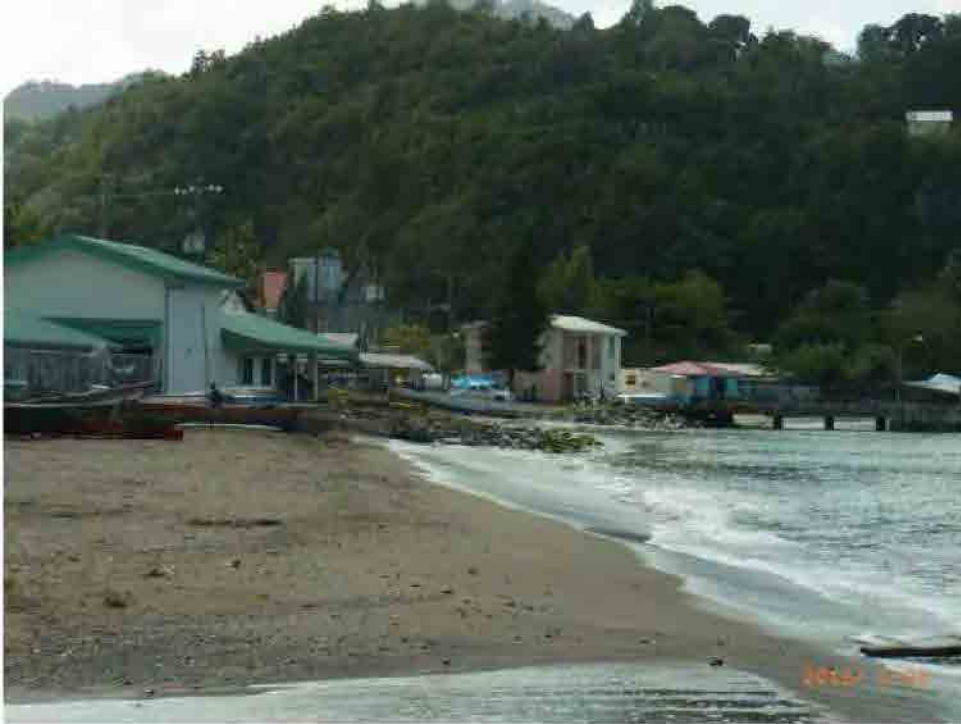
Photo 2-2-3-14 Armor stone part and foreshore slope in front of Fisheries Complex (1)
