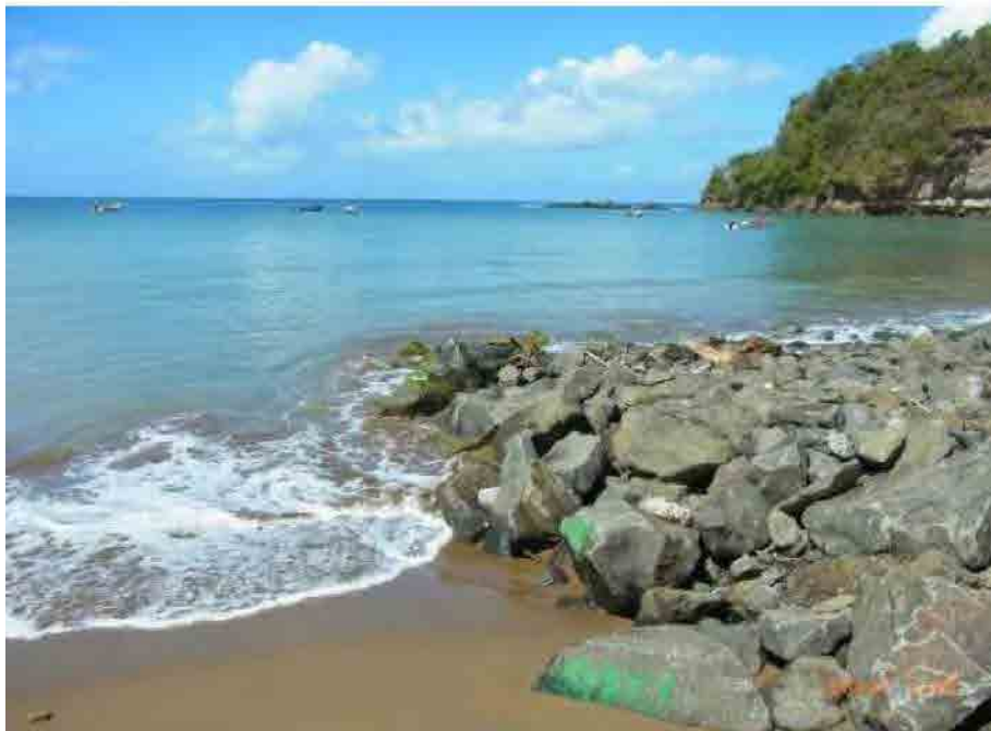
Photo 2-2-3-19 Foreshore side situation in front of Arcade at south side of armor stone part
