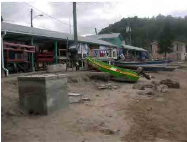
Photo-9 Foreshore condition of Vendors Arcade at one year inspection (2011/02/28)
