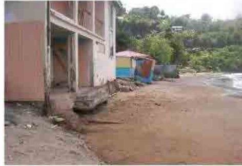
Beach situation in front of the Community Center at one year inspection (subsidence of 1m); Feb. 08, 2011
