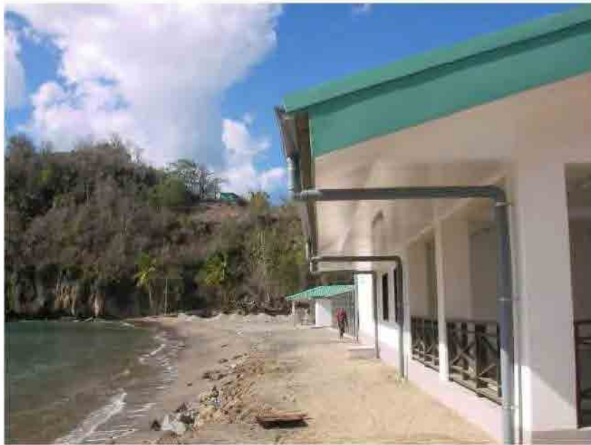
Feb. 19, 2010 at the completion of construction
