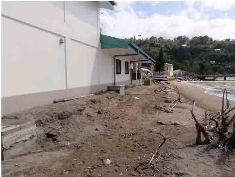
Feb. 08, 2011 at One year inspection
