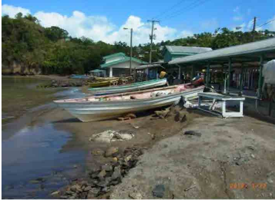
Photo 2-2-3-12 Armor stones situation in front of Arcade
