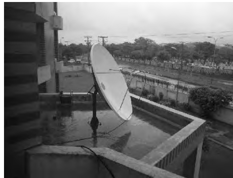
Receiving Antenna of Satellite Imagery by Feng Yun 2 at the PMD Head Office in Islamabad
