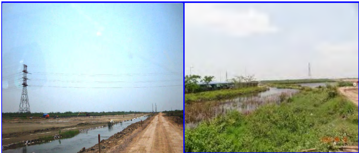
Photo: Ha Noi –Hai Phong Highway construction site
