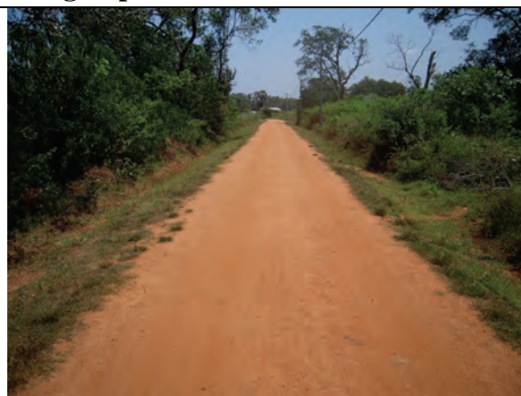
Final shape of Village Road at Vilathikulam, Madhu
