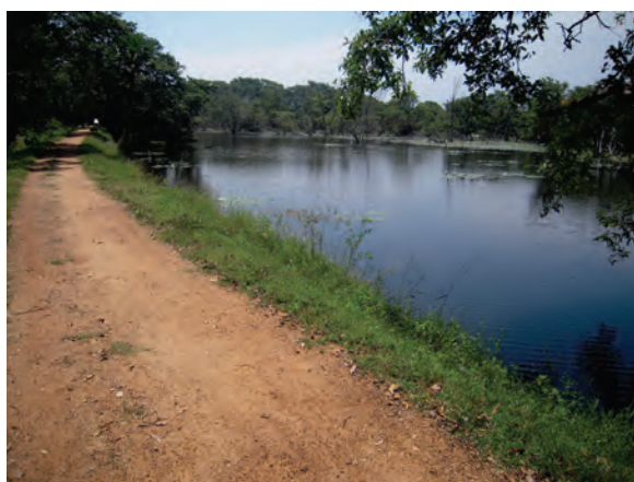
Final shape of renovated Irrigation Tank at Vilathikulam, Madhu
