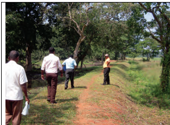
Final Inspection on Flood Dike at Cheddiyarmagan Kaddaiadampan, Nanaddan
