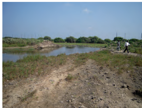
Breached tank bund due to the flood, which caused damages to the Village Road constructed by the Project at Theththavaady, Manthai West
