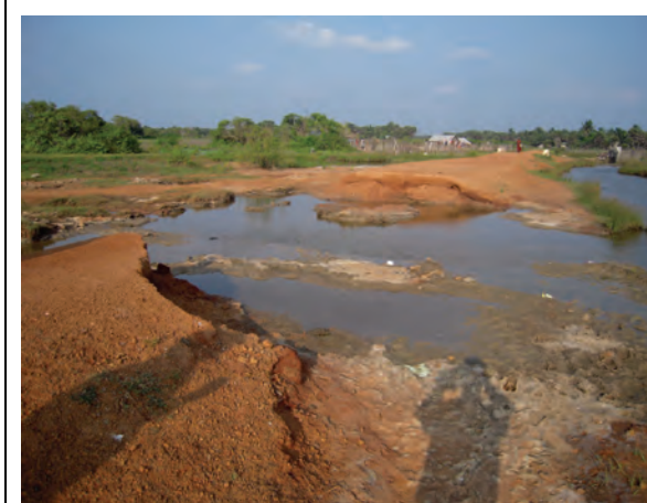
Village Road washed out by flood at Puthukadu, Manthai West
