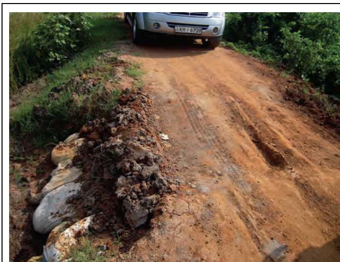
Chalampan Tank Bund Flood Release Cut
