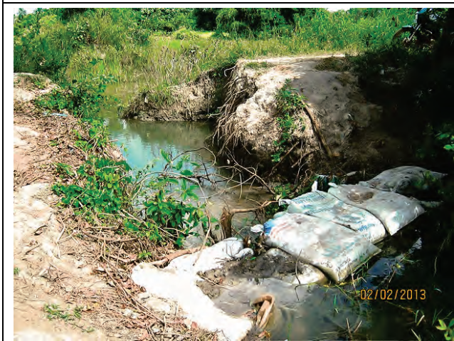
Katunkandal Tank Breached (Nedunkandal upper stream)
