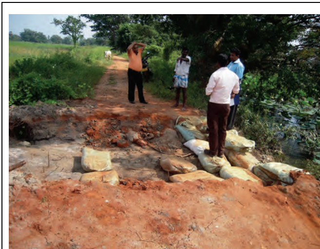
Nedunkandal Tank Cut to Release Flood (1)
