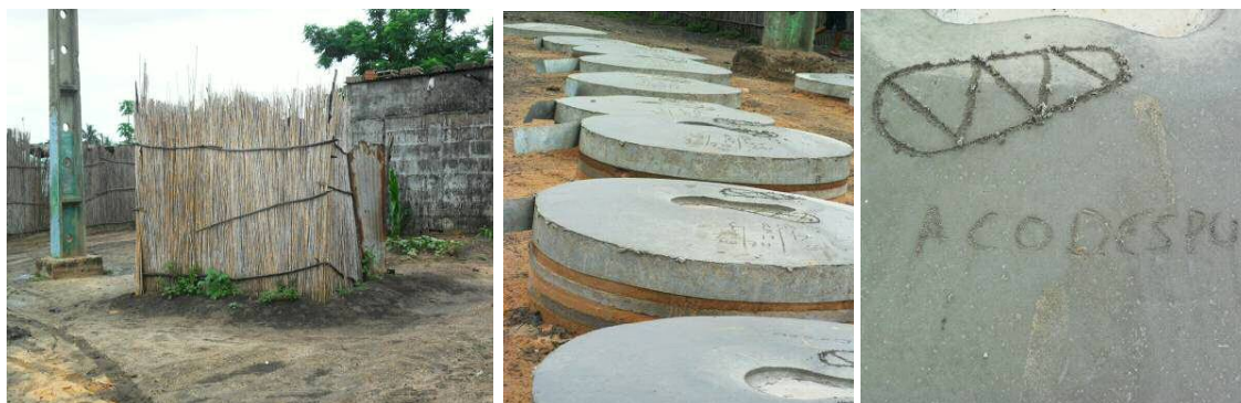
Figure 27: Traditional latrine in the project area; production of cement slabs by ACODESPU
