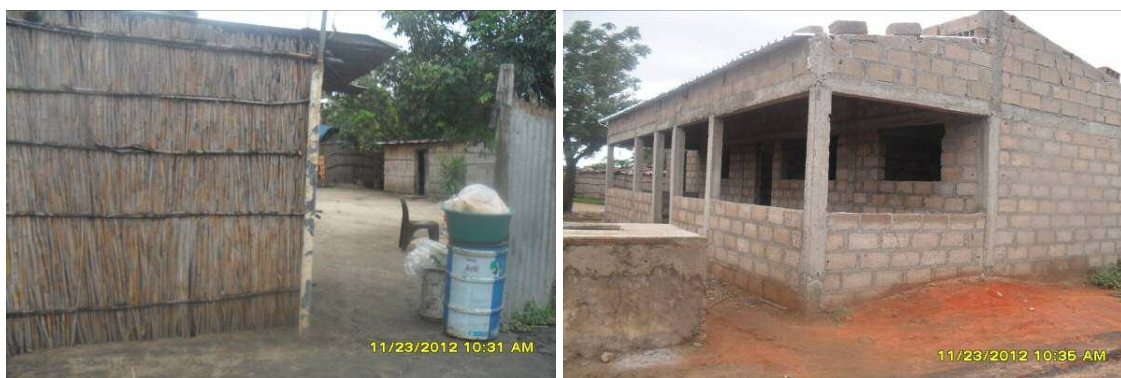
Figure 23: Reed and concrete houses in quarteirão 40a
