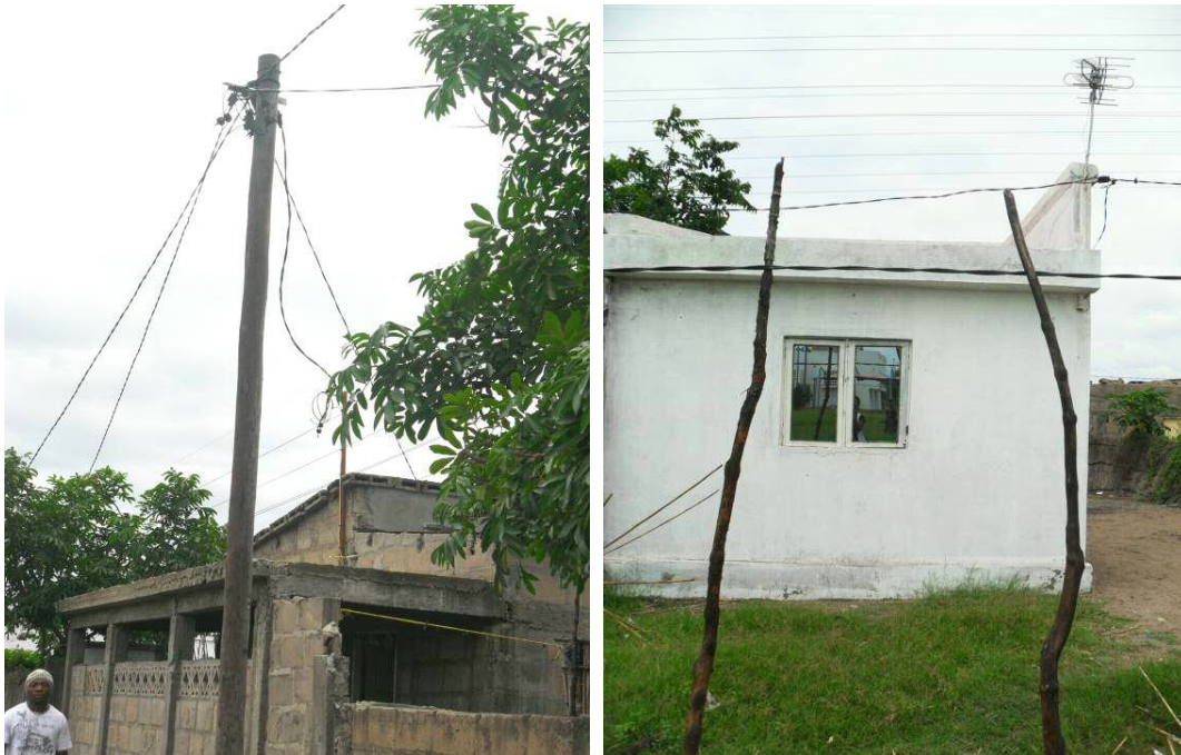
Figure 26: Electricity post and TV antenna in quarteirão 40a
