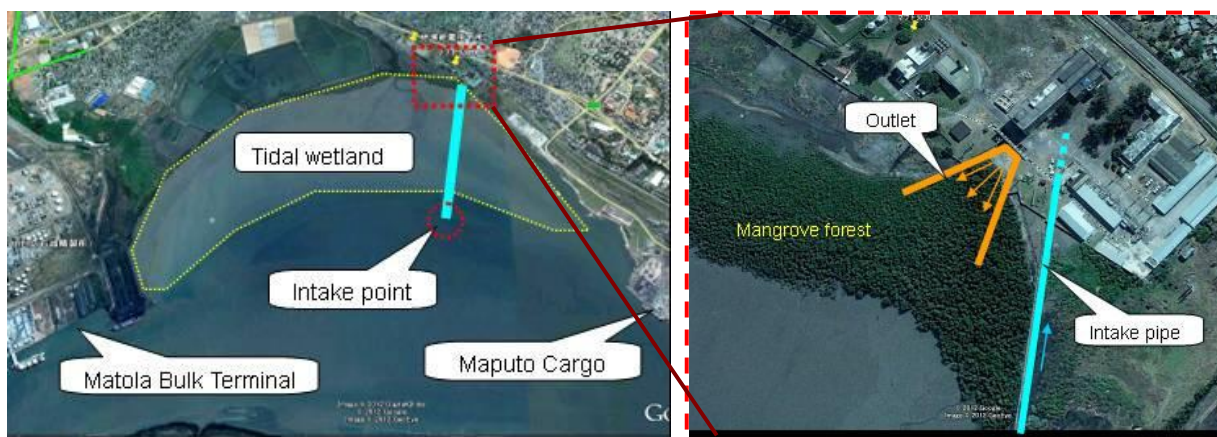
Water intake point of former coal fired power plant (complete view)
