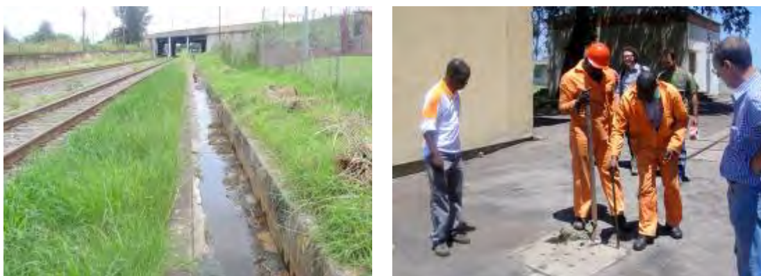
Figure 6.6-6 A drainage channel parallel to railway (70 cm wide) and a storm drain in CTM
