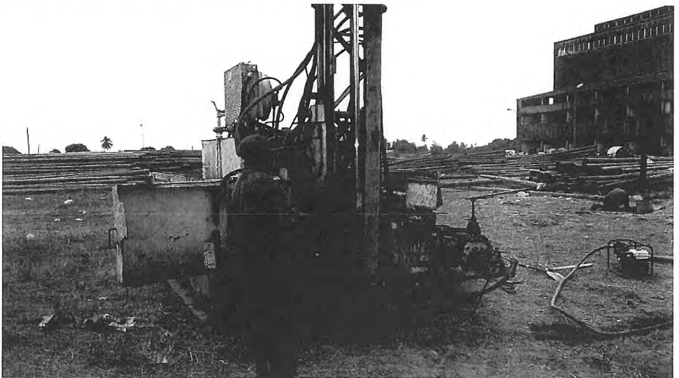
Plate B: Drilling Process at Test Location.
