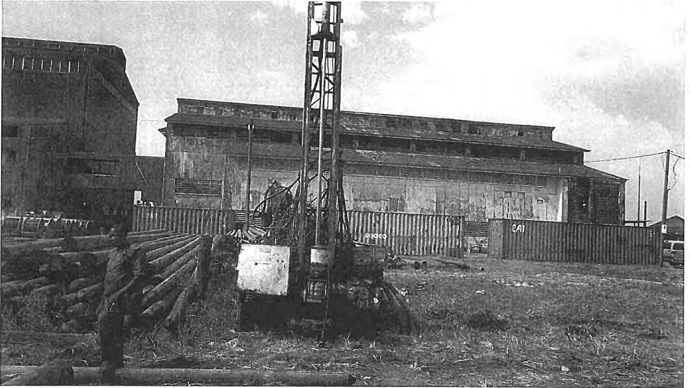
Plate A: Position of Rig at Test Location.
