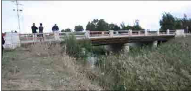
Figure 6.3-20 Current Status of GP8 Bridge and Road Over Mabtouh Bridge (Aug., 2012)
