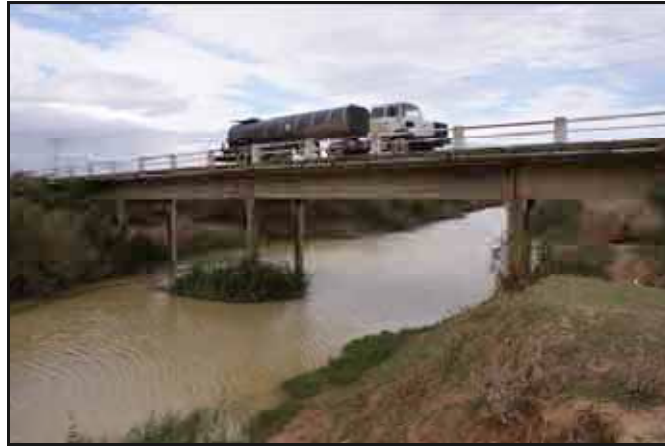
Figure 6.3-5 Current Status of GP8 Bridge Over Oued Mejerda Bridge (Aug., 2012)
