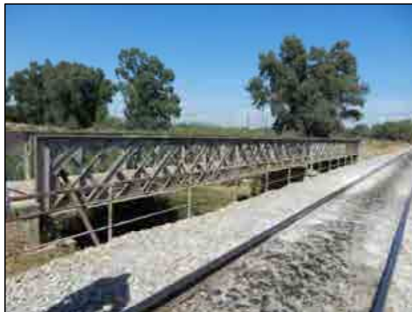
Figure 6.3-7 Current Status of Jedeida Railway Old Bridge (Aug., 2012)
