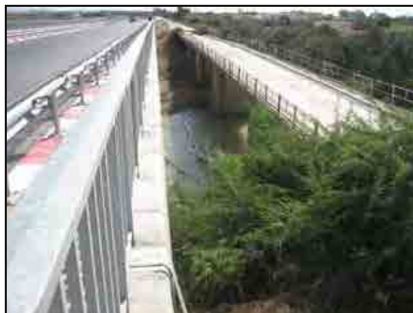
Figure 6.3-3 Tobias Old Bridge in August 2012
