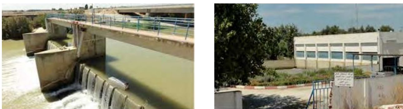
Figure 2-11: Left: Two tumble gates (in front) and the fixed dam/Right: Pumping station intake facilities directly upstream on the left bank
