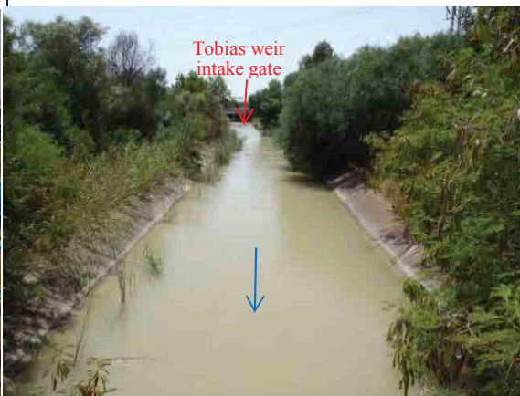
26. Water conduit from the Tobias weir (2012.08)
